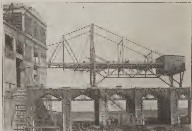
FIG 1. JUNCTION OF DAM AND POWER HOUSE.
