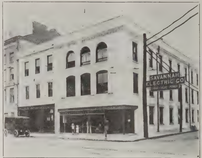
FIG. 8. VIEW SHOWING OFFICE OF SAVANNAH ELECTRIC COMPANY AND EDISON SUBSTATION AT LEFT.
