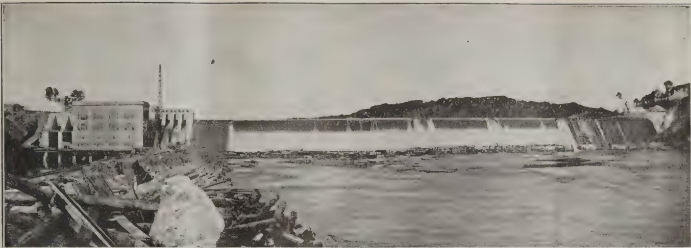
POWER HOUSE AND DAM OF GOAT ROCK HYDROELECTRIC DEVELOPMENT OF COLUMBUS POWER CO.
