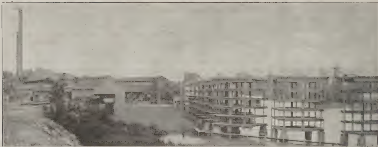
GENERAL VIEW OF PLANT OF ATLANTA STEEL COMPANY, ATLANTA, GA.
