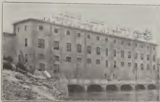
FIG. 2. BLEWITT STATION OF YADKIN RIVER POWER CO.
