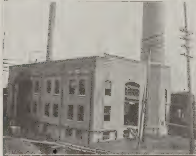
FIG. 1. NEW AUGUSTA STATION (WEST PLANT) SHOWING CONDENSER AT LEFT AND COAL TRESTLE AT RIGHT.
