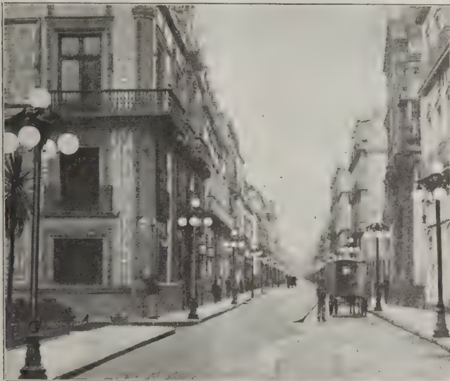
FIG. 1. AN INSTALLATION OF TUNGSTEN CLUSTERS IN MEXICO CITY, MEXICO.
