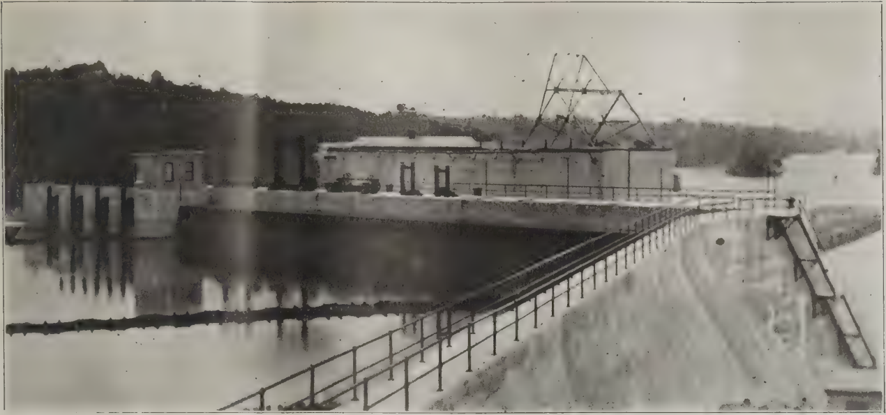
FIG. 16. VIEW OF UP-STREAM SIDE OF POWER STATION.
