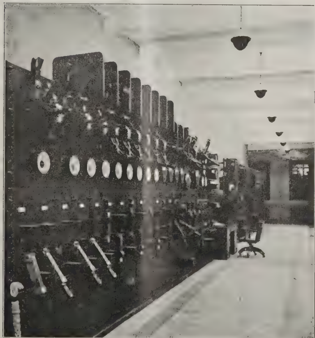
FIG. 1. VIEW IN SUBSTATION OF UNITED ELECTRIC LIGHT & POWER COMPANY USING INDIRECT LIGHTING.
