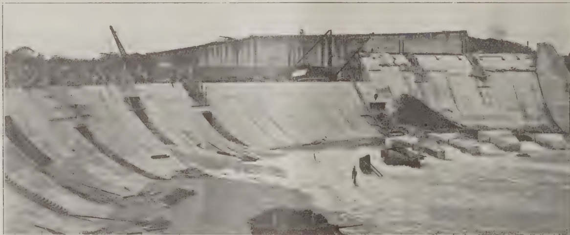
FIG. 3. THE GATUN SPILLWAY. VIEW LOOKING SOUTHWEST, SHOWING DOWN-STREAM FACE OF OGEE DAM.
