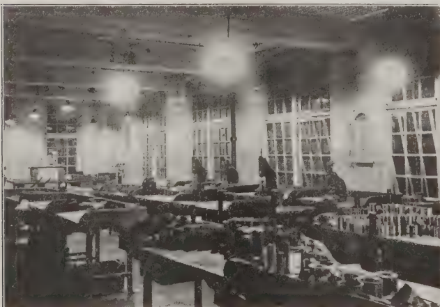
FIG. 4. NIGHT PHOTOGRAPH OF ILLUMINATION IN INSPECTION DEPARTMENT OF MANUFACTURING PLANT, SHOWING LOCALIZED GENERAL ILLUMINATION WITH BOWL SHAPED, PORCELAIN ENAMEL FINISHED, INTENSIVE, STEEL REFLECTORS AND 100-WATT TUNGSTEN LAMPS.
