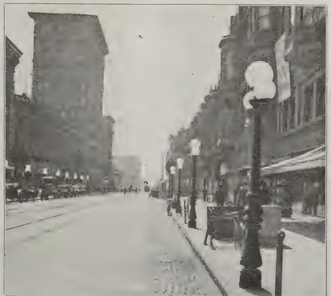
FIG. 2. AN INSTALLATION AT LOS ANGELES, CALIF., SHOWING POSITION OF THREE LIGHT POSTS.
