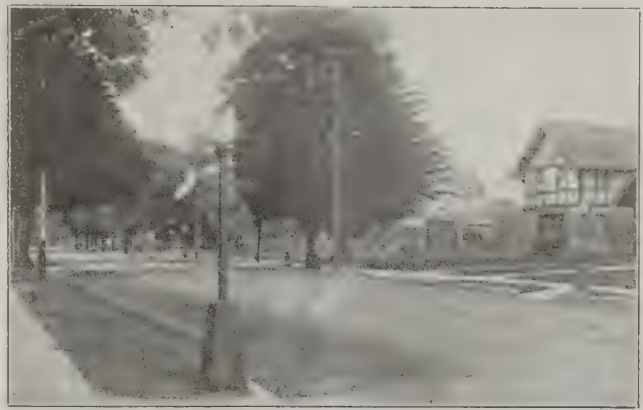
FIG. 5. A TYPICAL STREET VIEW AT ALAMEDA, CALIFORNIA, shown at the right of Fig. 3 is an excellent unit for such lighting in boulevard driveways, automobile courses, etc. It gives an extended light distribution having a reflector above the arc, and is mounted at a height of 18 feet, well above the line of vision. This lamp is especially applicable to wide parkways where the lighting is not influenced by the presence of trees. There is another luminous lamp very similar in appearance and design to the ornamental type used in Baltimore known as the residential type. This lamp is mounted at a height of fourteen feet and may be placed below the foliage lining residence streets. Diffusing globes are used so that there is no apparent glare.
