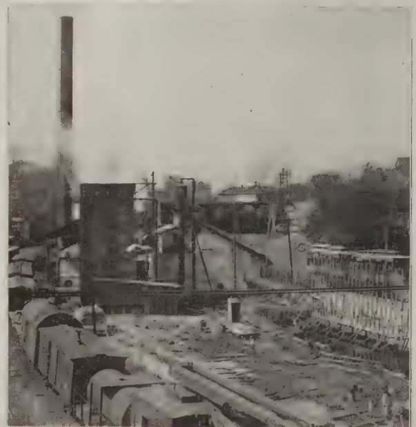
FIG. 2. GENERAL VIEW OF PROPERTY BEFORE RECONSTRUCTION.
