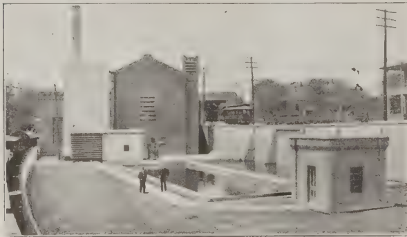
FIG. 1. GENERAL VIEW PRESENT POWER PLANT VICKSBURG LIGHT AND TRACTION COMPANY.
