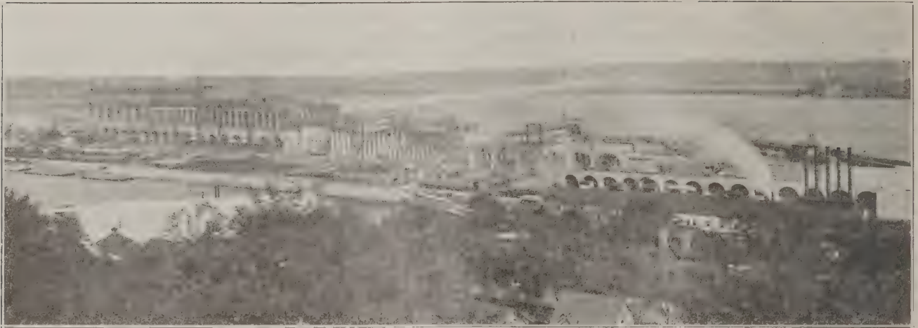
A GENERAL VIEW OF LOCK, POWER HOUSE AND DAM OF THE MISSISSIPPI RIVER POWER COMPANY'S DEVELOPMENT.
