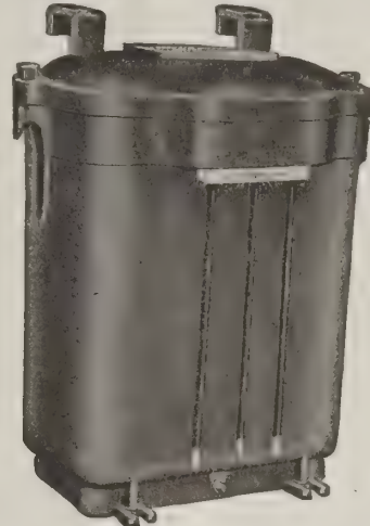
FIG. 2. THREE-PHASE SINGLE UNIT TRANSFORMER.
