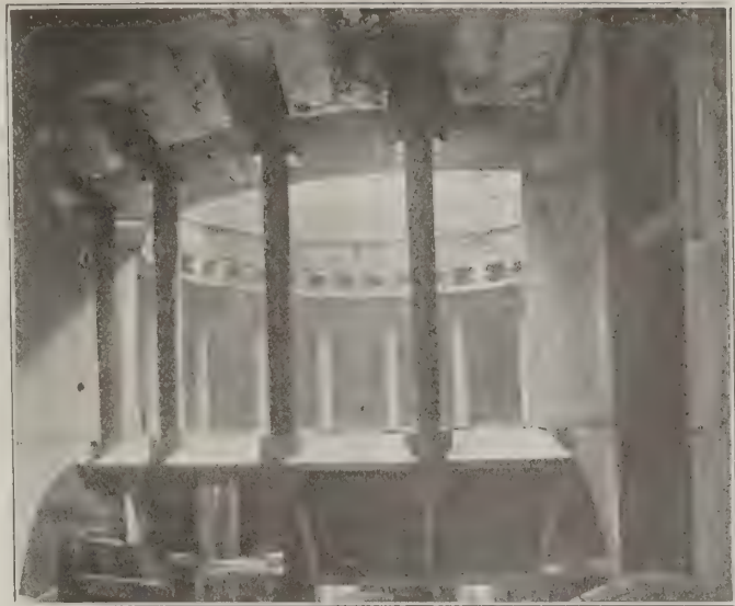
FIG. 2. WHEEL CHAMBER SHOWING BOLTS AND BAFFLE PLATES.
