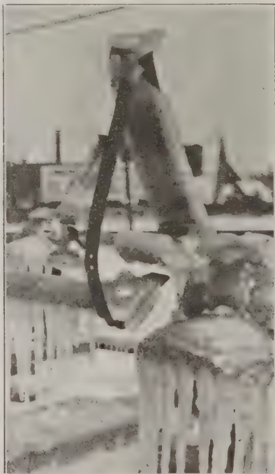
FIG. 2. SHOWING ACTION OF CONTACTS BREAKING ICE.
