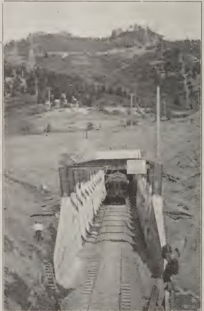
FIG. 2. SHEPARD'S CANYON TUNNEL THROUGH CONTRA COSTA HILLS.
