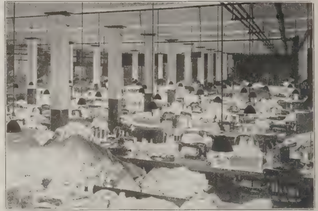
FIG. 5. NIGHT PHOTOGRAPH OF THE FINISHING DEPARTMENT OF A KNITTING MILL, SHOWING LOCALIZED ILLUMINATION WITH DEEP BOWL, ALUMINUM FINISHED, FOCUSING STEEL REFLECTORS AND 25-WATT TUNGSTEN LAMPS.
