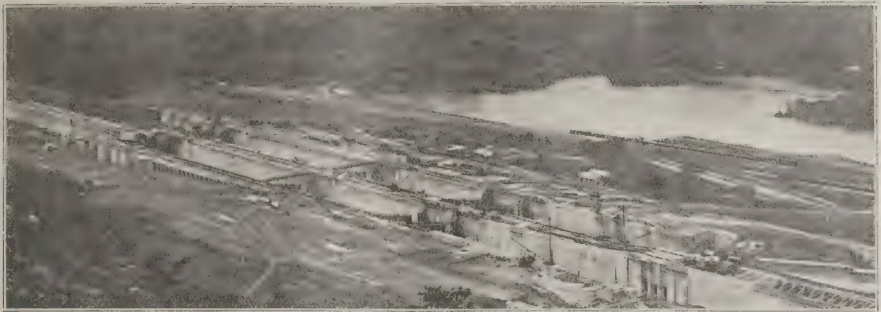
FIG. 4. THE PEDRO MIGUEL LOCKS. BIRDSEYE VIEW FROM HILL ON EAST BANK.—JULY 28, 1912.
