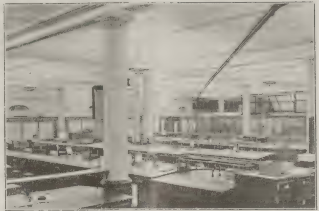
FIG. 20. NIGHT PHOTOGRAPH OF THE ILLUMINATION IN THE ACCOUNTING DEPARTMENT, SHOWING THE GENERAL ILLUMINATION WITH PORCELAIN ENAMELED, SINGLE UNIT, TOTALLY INDIRECT LIGHTING FIXTURES AND 400-WATT TUNGSTEN LAMPS.
