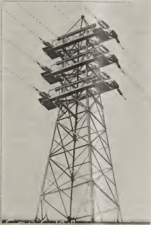
FIG. 11. RIVER CROSSING TOWER AT CHATTANOOGA.
