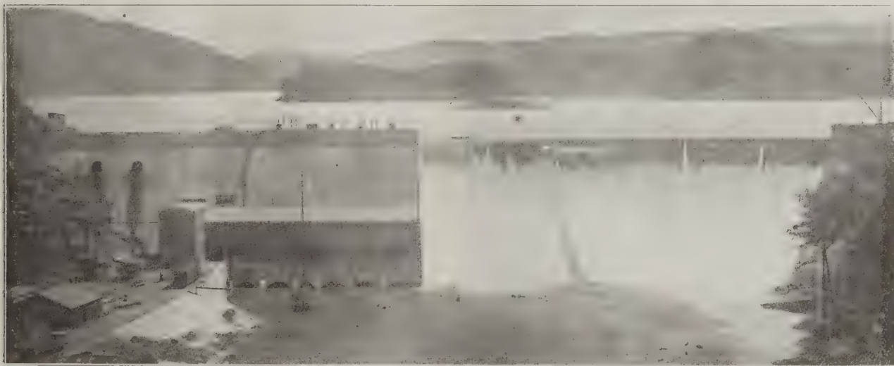
FIG. 1. VIEW OF DAM AND POWER HOUSE, LOOKING UPSTREAM.
