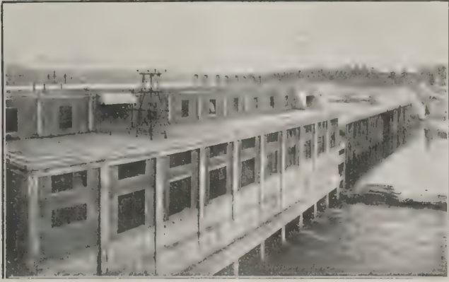
FIG. 1. DOWN-STREAM SIDE OF POWER HOUSE AND DAM. walls and dam show no leakage under pressure of the fifty foot head. Most of the timber used for building coffer-dams and other temporary structures was obtained by clearing the land to be submerged by the lake.
