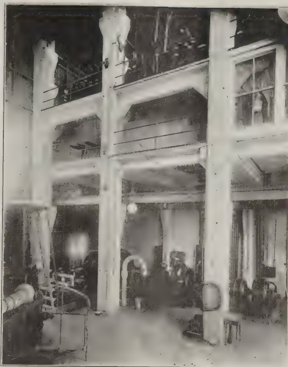
FIG. 6. VIEW OF STEAM STATION SHOWING SWITCHBOARD GALLERY.
