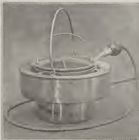
FIG. 2. ELECTRIC GLUE POT.
