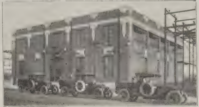
FIG. 10. JOPLIN SUB-STATION, SHOWING 33,000-VOLT ENTRANCES.
