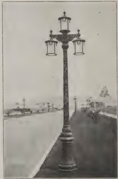
FIG. 7. AN INSTALLATION OF ORNAMENTAL POSTS AT WINDSOR SQUARE, LOS ANGELES, CALIFORNIA, USING ALBA GLASS CYLINDERS.
