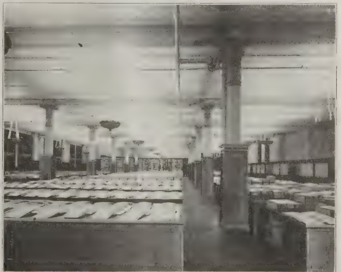
FIG. 9. ILLUMINATION DISPLAY ROOM WM. MEYER AND COMPANY, NEW YORK CITY.
