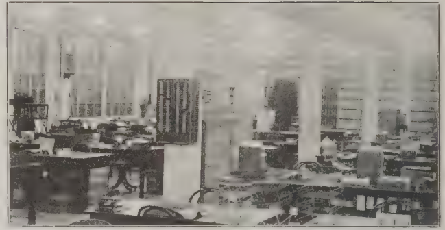
FIG. 16. NIGHT PHOTOGRAPH OF ILLUMINATION IN A CLERICAL OFFICE, SHOWING GENERAL ILLUMINATION WITH BOWL-SHAPED PRISMATIC CLEAR REFLECTORS AND 100-WATT TUNGSTEN LAMPS.
