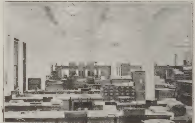
FIG. 18. NIGHT PHOTOGRAPH OF THE ILLUMINATION IN A GENERAL OFFICE, SHOWING GENERAL ILLUMINATION WITH LEADED GLASS, SEMI-INDIRECT LIGHTING UNITS AND 250-WATT TUNGSTEN LAMPS.
