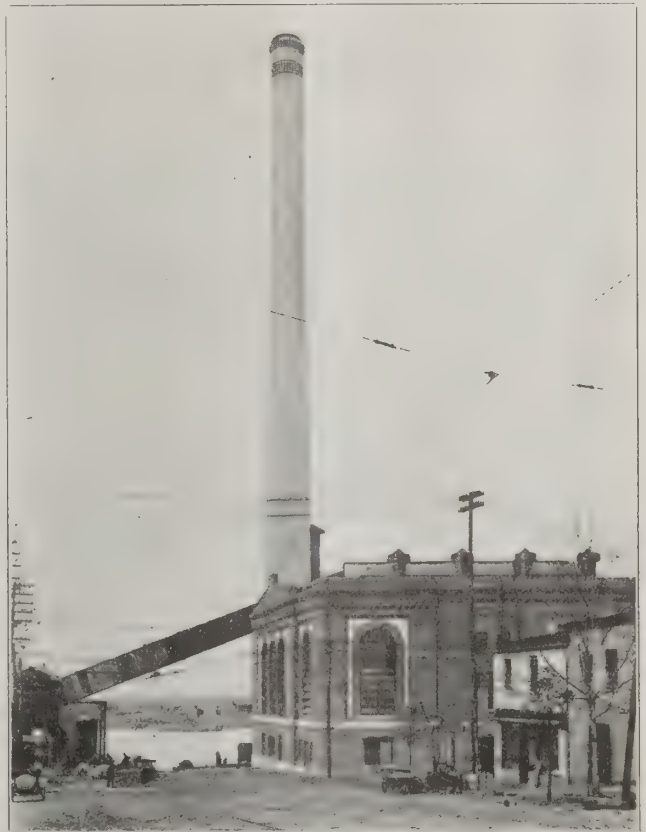
FIG. 1. RIVERSIDE STATION (SAVANNAH) SHOWING COAL STORAGE AND CONVEYOR.
