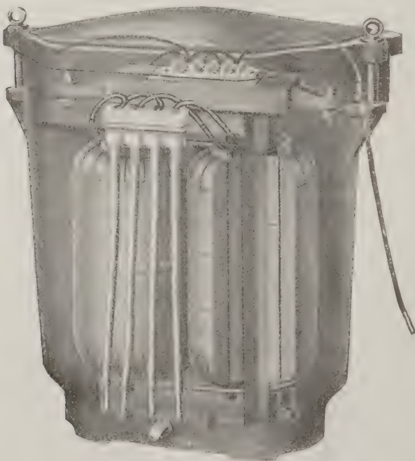
FIG. 1. CONSTRUCTION DETAILS OF PACKARD TRANSFORMERS.
