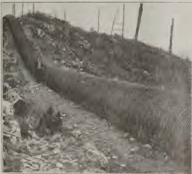
FIG. 2. PIPE LINE TO GENERATING STATION.
