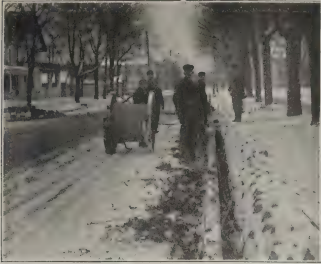
FIG. 2. LAYING STEEL TAPED CABLE IN PARKWAY, KENDALLVILL, IND.
