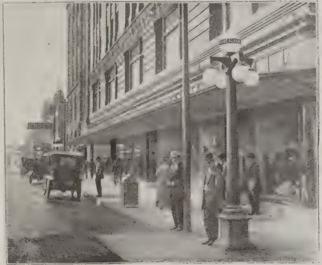
FIG. 9. AN APPLICATION OF FIRE ALARM GLOBES AT FORT WORTH, TEXAS.
