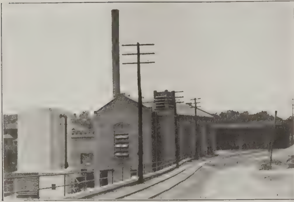
FIG. 5. VIEW SHOWING POWER PLANT AND CAR BARN.
