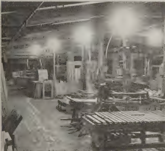
FIG. 7. NIGHT PHOTOGRAPH OF WOOD-WORKING SHOP, SHOWING LOCALIZED-GENERAL ILLUMINATION WITH PORCELAIN ENAMELED, FLAT DOME TYPE, STEEL REFLECTORS AND 250-WATT TUNGSTEN LAMPS.
