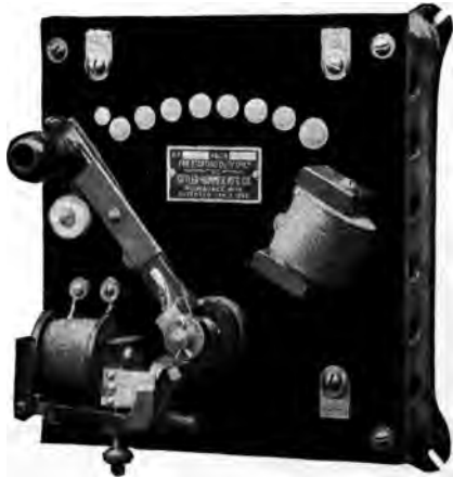
FIG. 225.—Cutler Hammer Starting Box.
