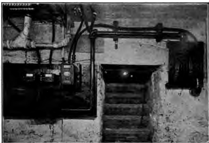
FIG. 303. — Typical Service of Meters.
