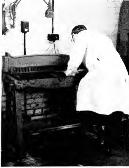
Plate 27.1 Foot-operated 3 ft. guillotine
