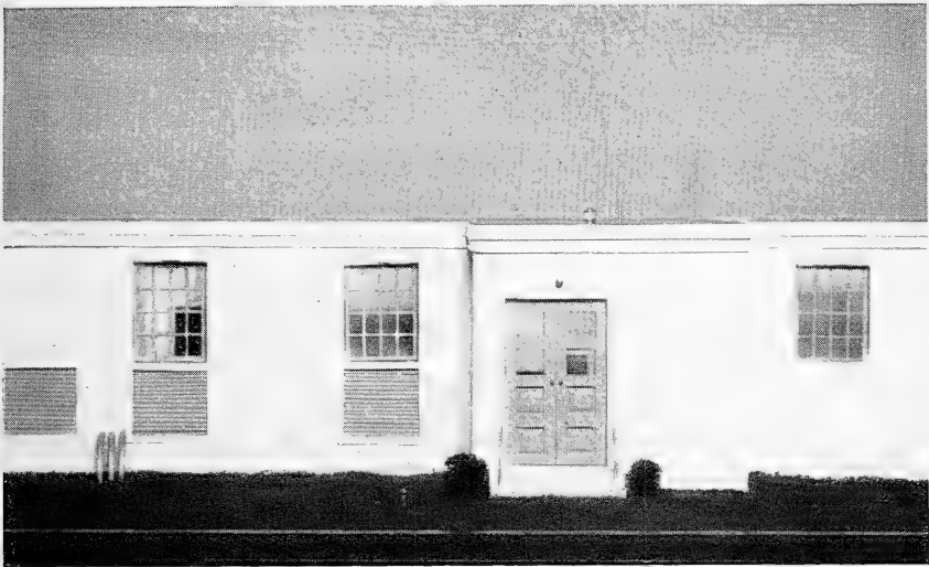
FIGURE 1-13.—Loran signal building.
