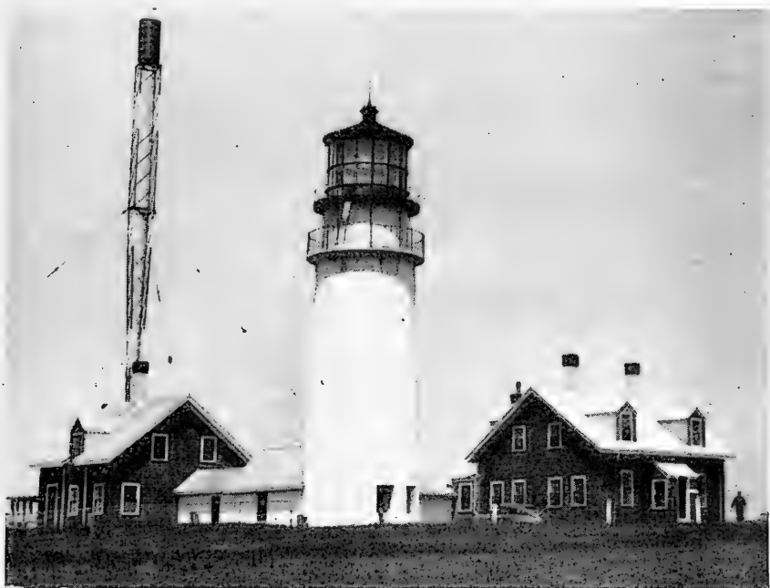
FIGURE 2-1.—Cape Cod Light Station, Massachusetts. Established 1798. Rebuilt 1857. Top of lantern 66 feet above ground. Light 183 feet above water. Foundation: rubble stone masonry. Signals: First order electric apparatus. Flashing white every 5 seconds. Flash 0.2 second, eclipse 4.8 seconds. 13,000 candlepower. High-power class A radiobeacon. Special antenna in background. Fog signal: horn, diaphragm, electric; blast 3 seconds, silent 12 seconds.
