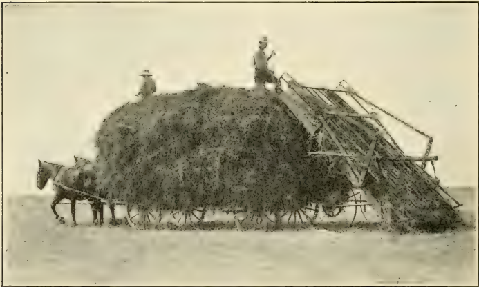
Figure 46.—A modern hay loader saves time and labor.
