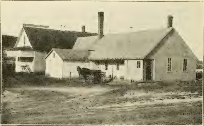
Figure 128.—A co-operative laundry in connection with a co-operative creamery.
