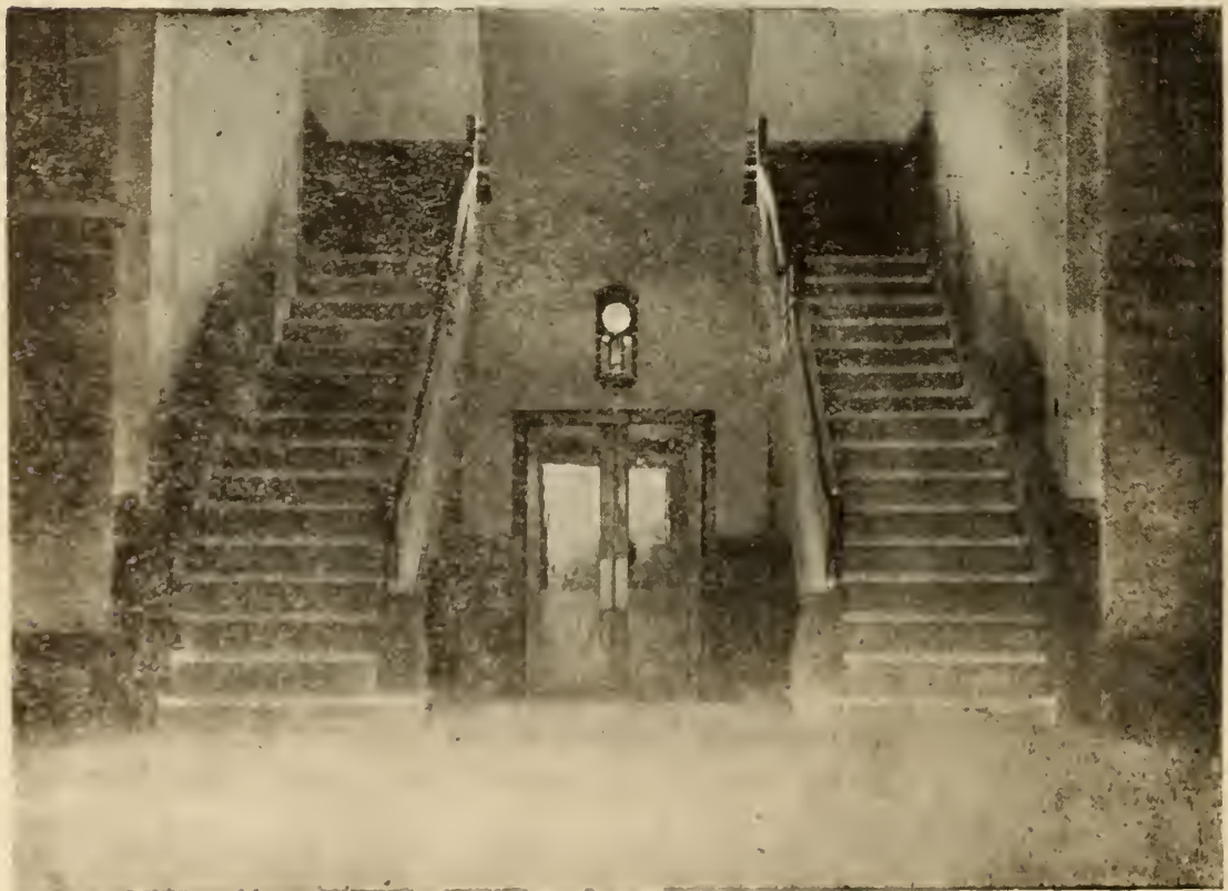
Stairway and Southern Exit
