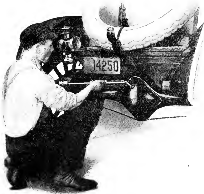
Pouring oil into the differential housing.
