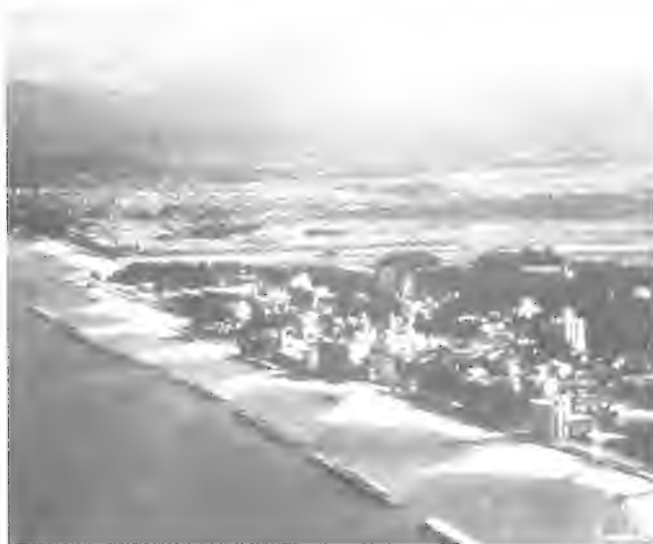
Figure 4. Segmented detached breakwaters in Japan
