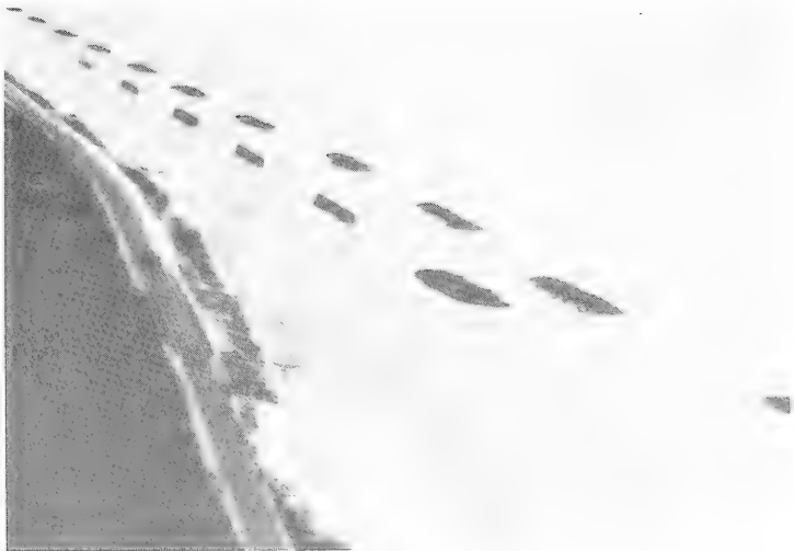
Figure 18. Segmented detached breakwaters near Peveto Beach, Louisiana
