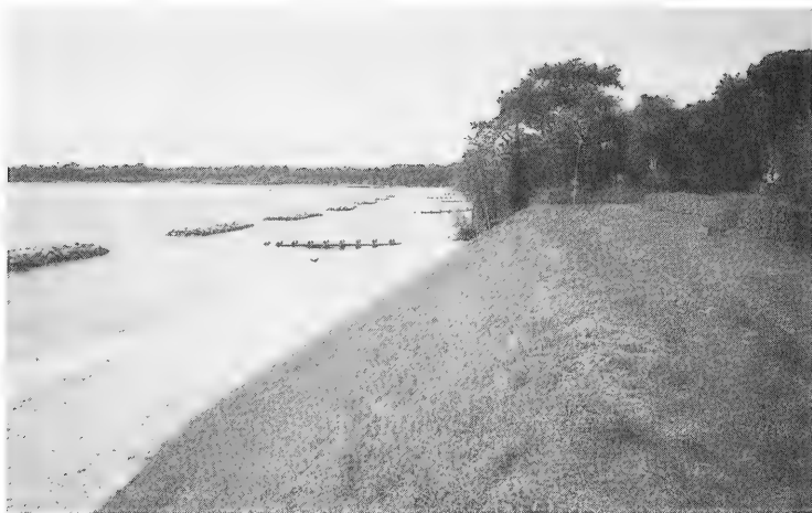
Figure A7. Completed project at south end
