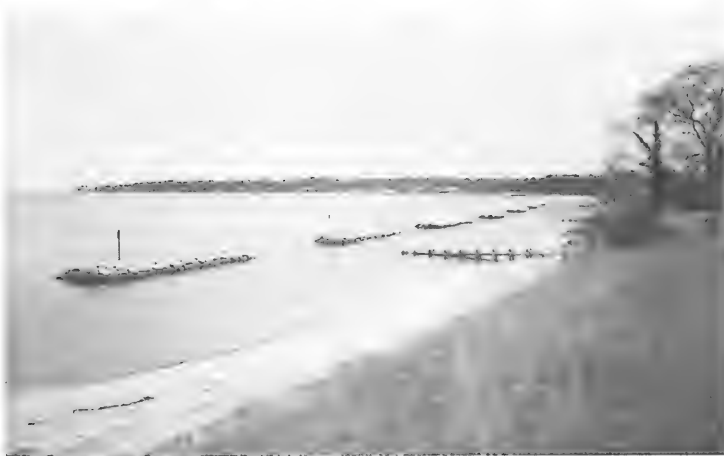
Figure 7. Detached breakwaters constructed on Chesapeake Bay at Bay Ridge, Maryland
