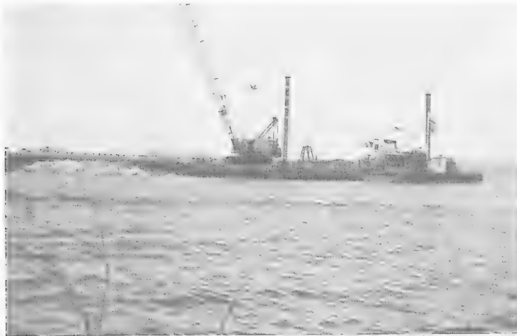
Figure 60. Breakwater 22 under construction at Presque Isle, Pennsylvania
