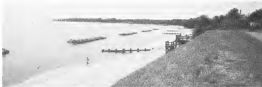
Figure A8. Completed project at north end
