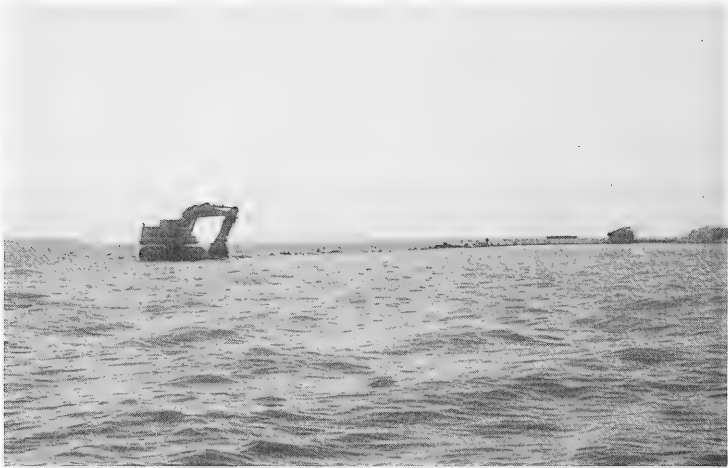
Figure 61. Land-based construction at Eastern Neck, Chesapeake Bay, Maryland
