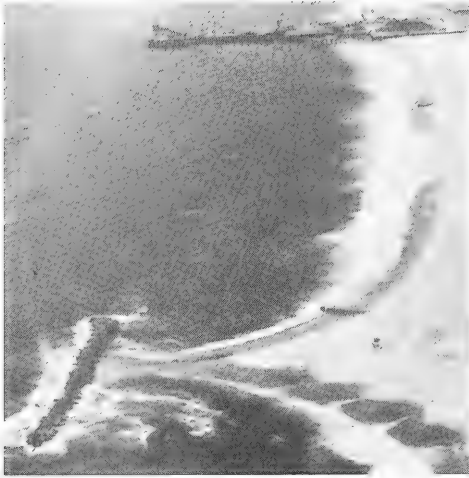
Figure 17. Single detached breakwater at Venice Beach, California
