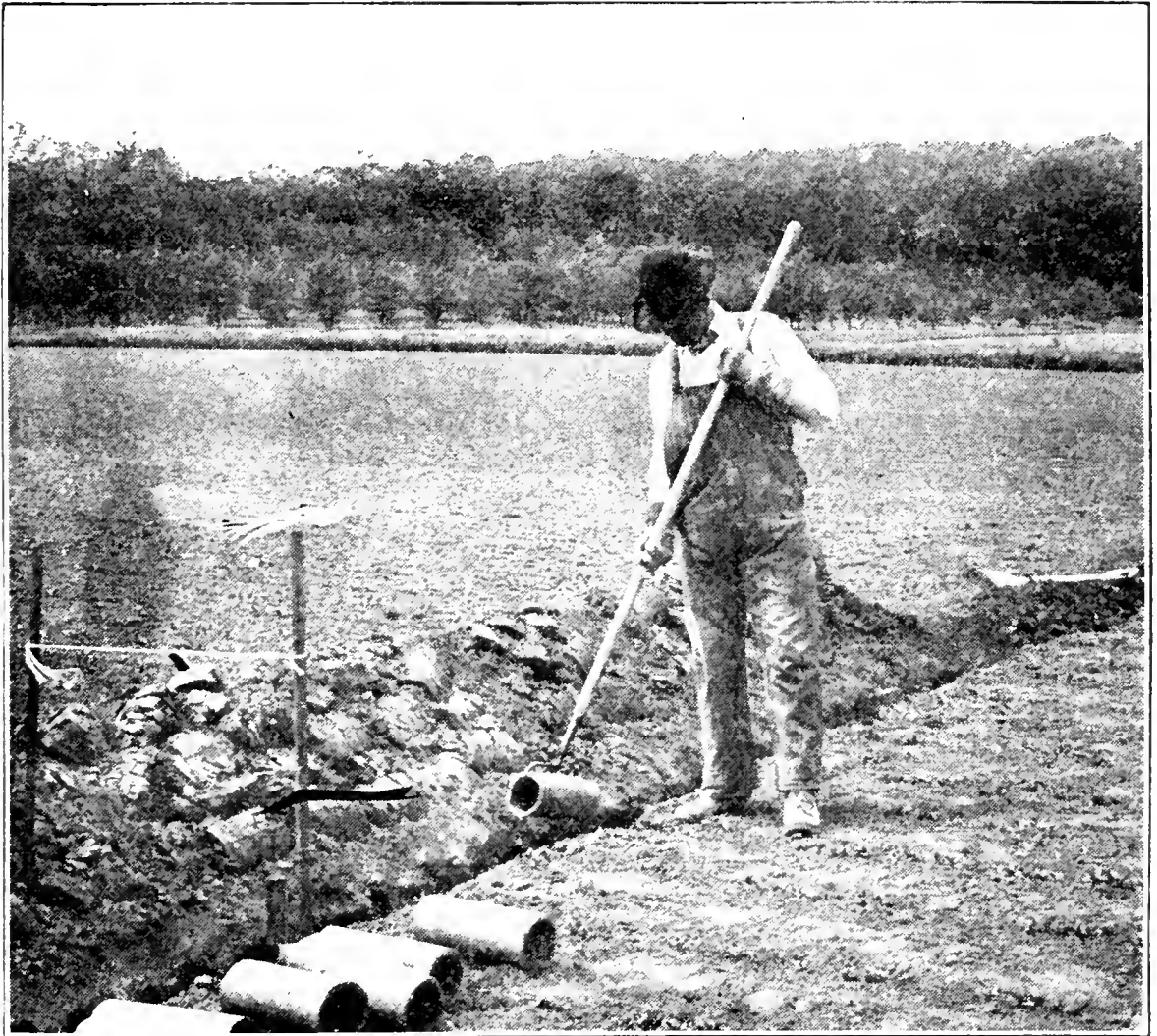
FIG. 238. Laying tile with a tile hook
