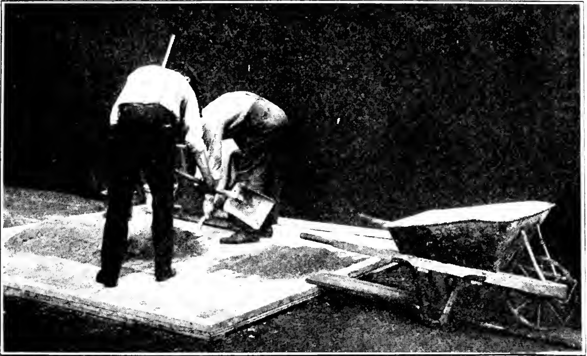
FIG. 137. Use of a mixing platform
