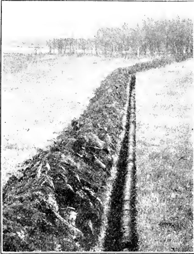
FIG. 239. Tile laid in trench ready for blinding
