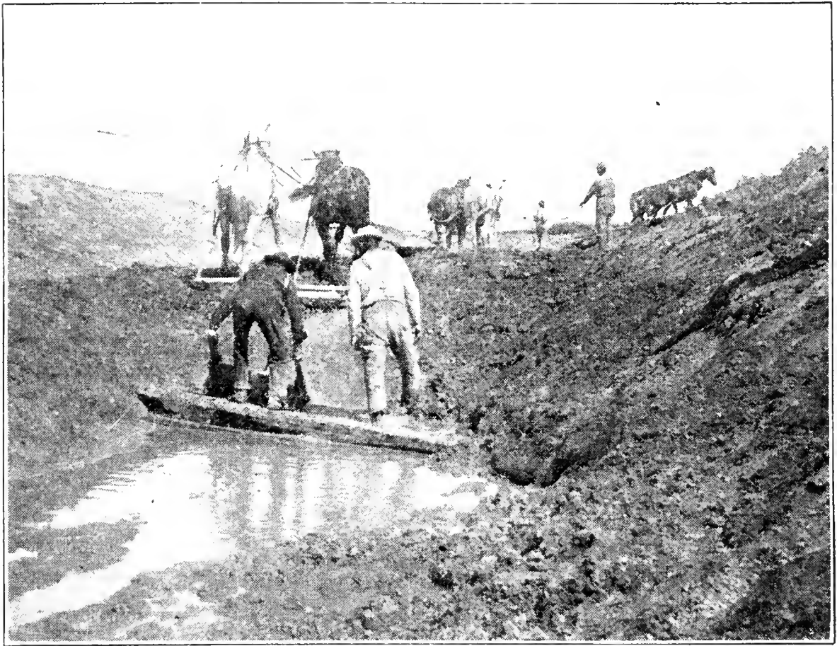
FIG. 228. Construction of an open ditch 10 feet deep by means of slip scrapers
