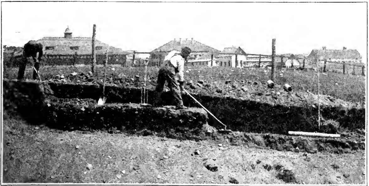
FIG. 235. Excavating a 3-foot tile trench
