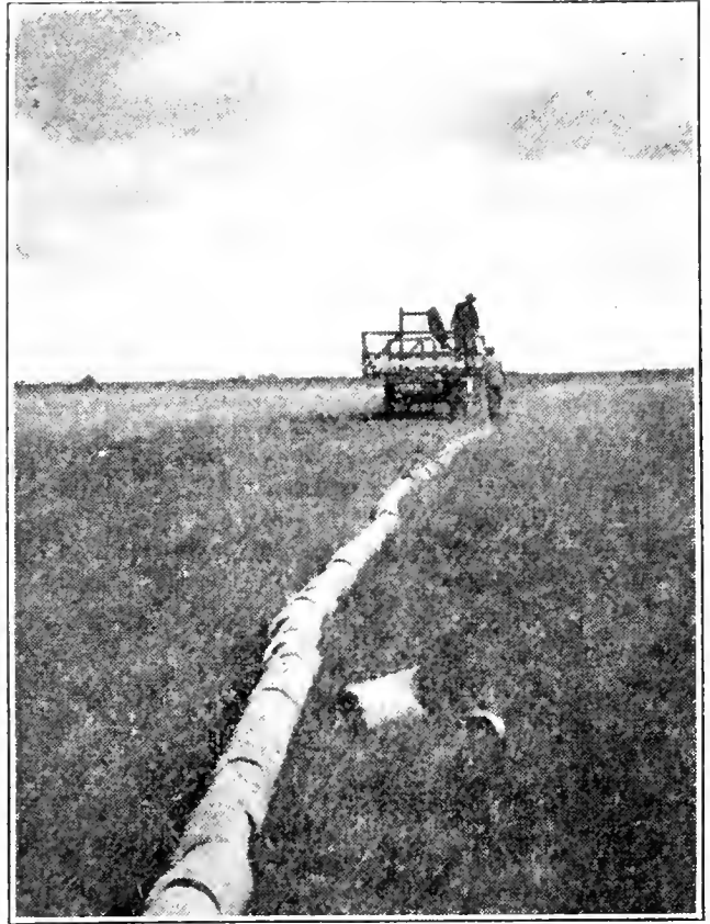
FIG. 233. Distributing tile on the line of trench
