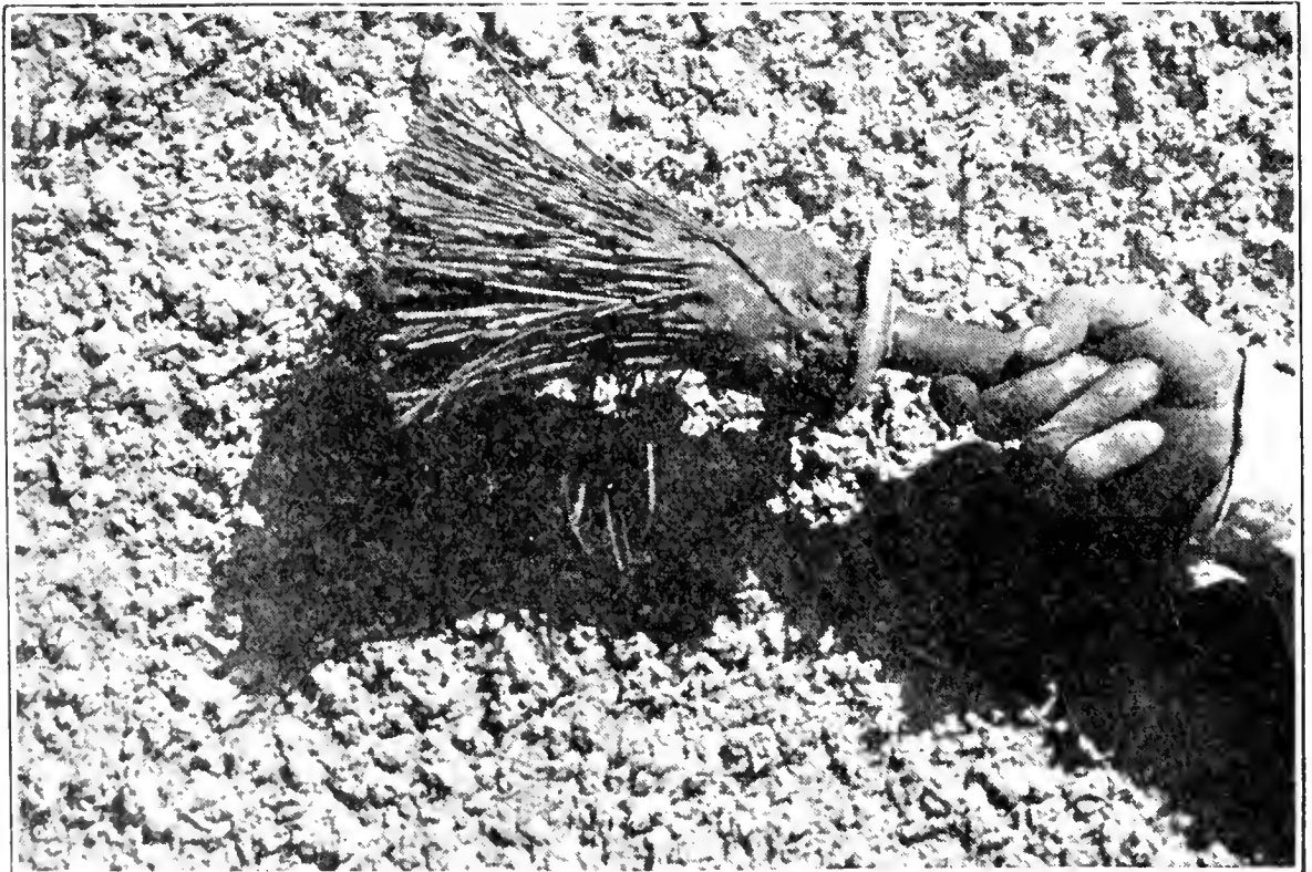
FIG. 151. Method of applying spatter coat
