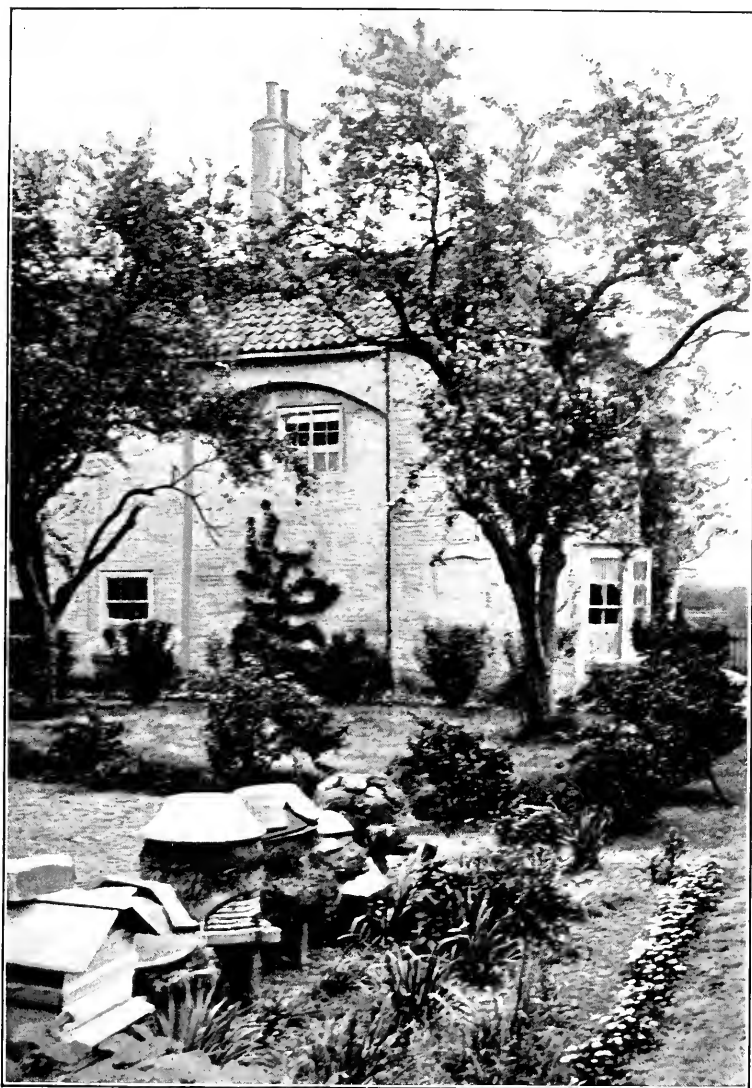
WEST SIDE OF MANOR-HOUSE
