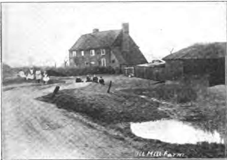
OIL MILL FARM.
