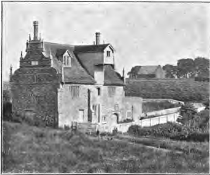
ST. JOHN'S ABBEY MILL, BOURNE POND.
