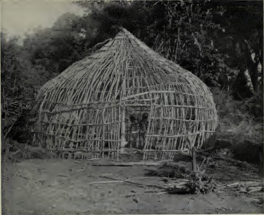
(22) Framework of a Kamba hut in course of construction.
