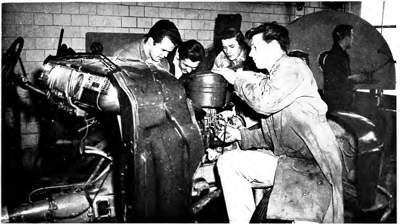
Four young Euclid mechanics take the first steps in dismantling a carburetor.
