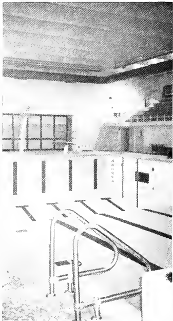
With the new dehumidifier installed in the boy's and girl's pools there should be less damage to the paint and walls.
