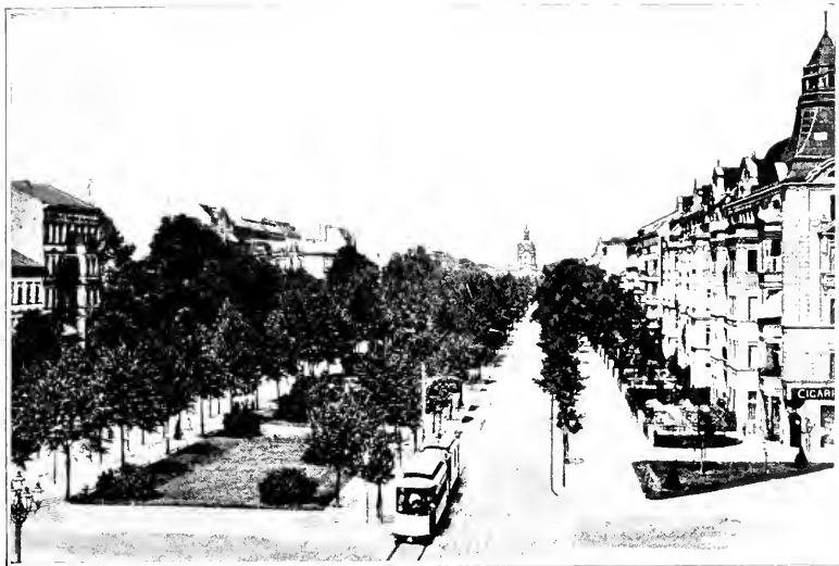
SPACIOUS STREET CONSTRUCTION, CHARLOTTENBURG.
