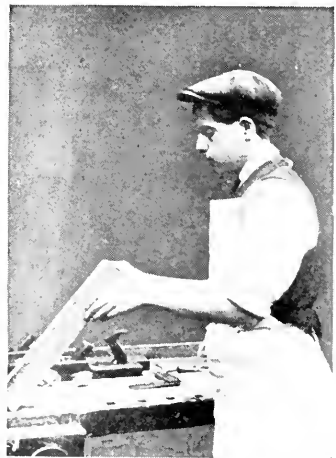
Sighting a Piece of Planed Wood for Straightness
