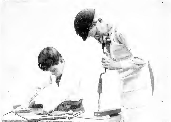
Removing Damaged Screw with Spanner
