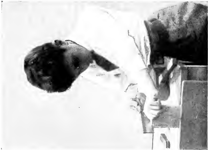
Cutting Dovetails with Dovetail Saw
