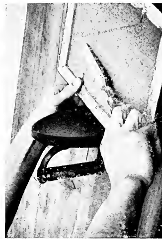
Driving in Sprigs with Old Chisel
