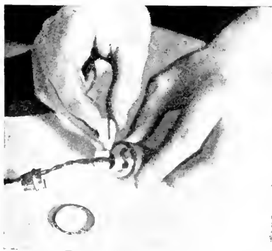
Fixing Cord Grip of Lamp Holder
