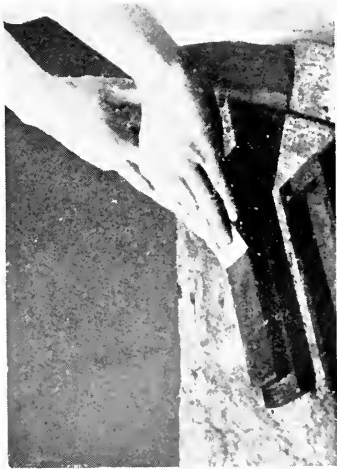
Sharpening a Plane Iron
