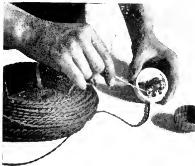
Wiring-up a Wall Switch
