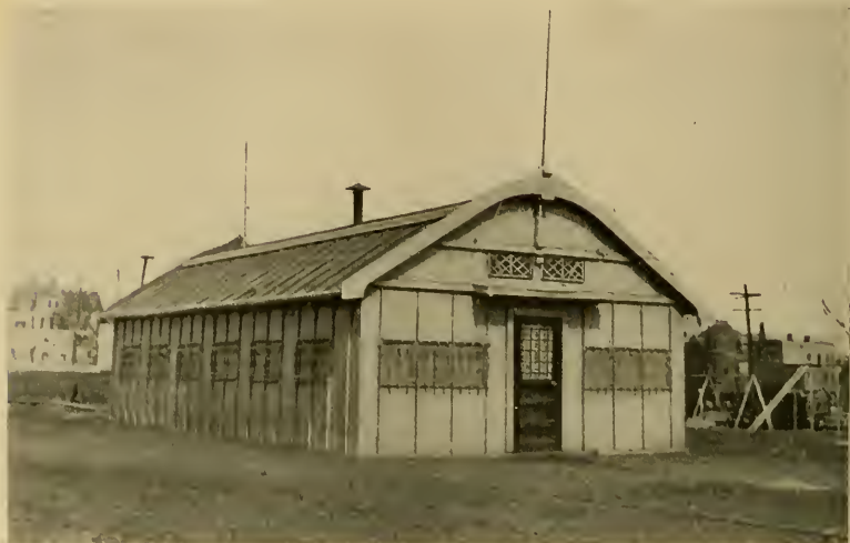
1 Fig. 111.—A portable steel recreation house, 20 by 40 ft., divided into two parts for boys and girls by a removable partition. Comfort stations, 12 by 12 ft., of similar construction, are divided into four sections containing two toilets and two shower baths (Newark Playground Commission Report, 1913).
