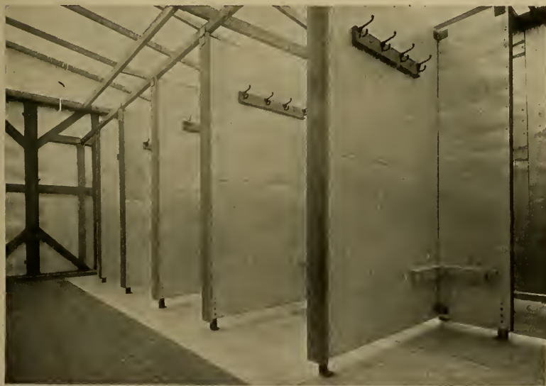
Fig. 113.—Portable bath-house used in Baltimore, Md. The inside (courtesy of Playground Association of America).
