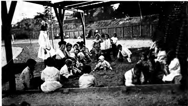
Fig. 108.—Sand pile (Waterview Park, Germantown, Pa.).
