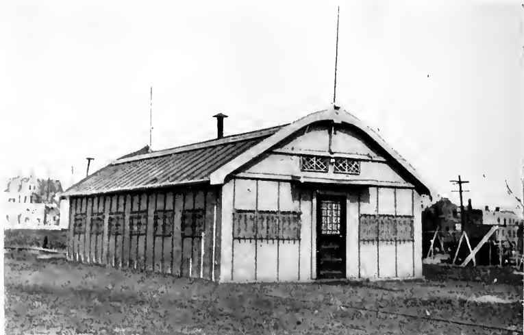
Fig. 111.—A portable steel recreation house, 20 by 40 ft., divided into two parts for boys and girls by a removable partition. Comfort stations, 12 by 12 ft., of similar construction, are divided into four sections containing two toilets and two shower baths (Newark Playground Commission Report, 1913).
