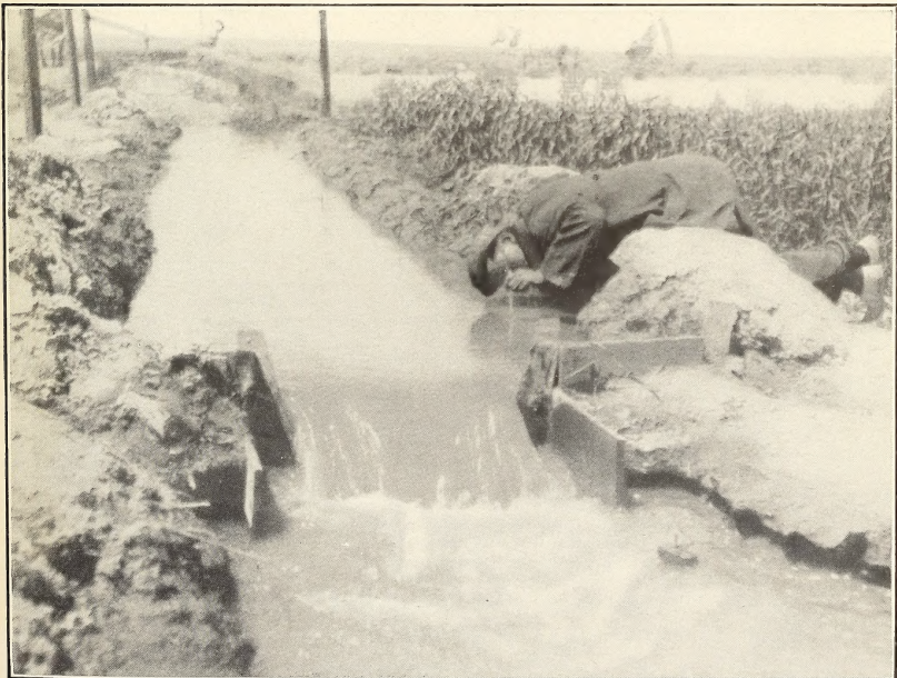
FIG. 2.—DOWNSTREAM VIEW OF CIPOLLETTI WEIR USED IN IDAHO INVESTIGATION, SHOWING METHOD OF MEASURING.
