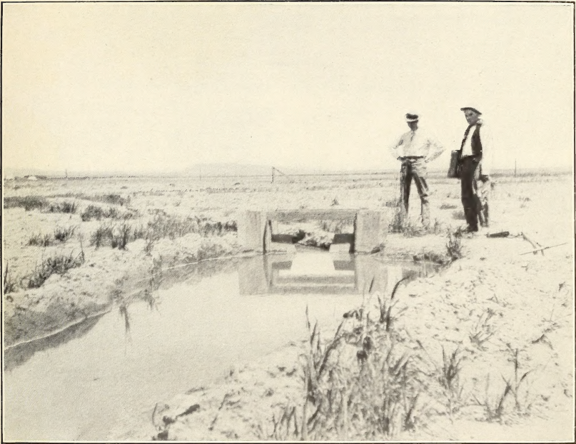
FIG. 1.—UPSTREAM VIEW OF CIPOLLETTI WEIR USED IN THE IDAHO INVESTIGATION.
