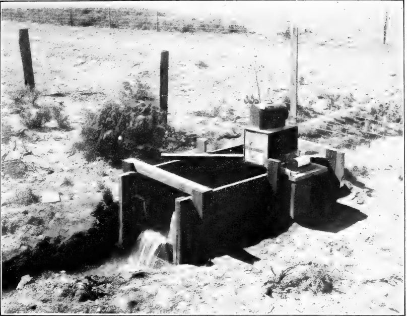
FIG. 1.—TYPE OF WATER REGISTER USED IN THE IDAHO INVESTIGATION, SHOWING THE METHOD OF INSTALLATION.
