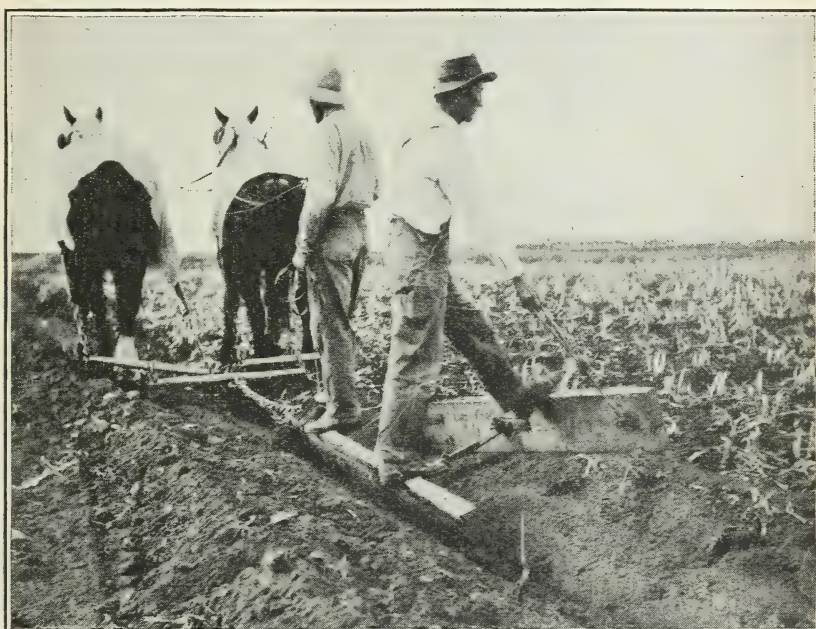
FIG. 15.—Constructing an irrigation ditch on the Belle Fourche Experiment Farm. The corn ground is irrigated before sowing it to winter wheat.
