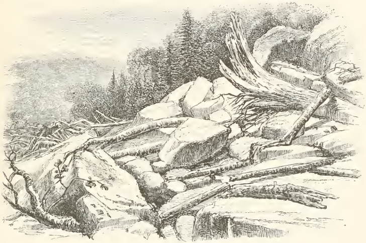
LAND-SLIDE ON COLD-WATER RIVER PORTAGE.
