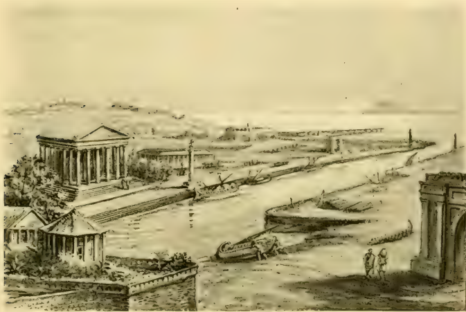
FIG. 21.—Puzzuoli or Puteoli in the time of the Roman Empire (third century). The dock and public buildings are represented.
