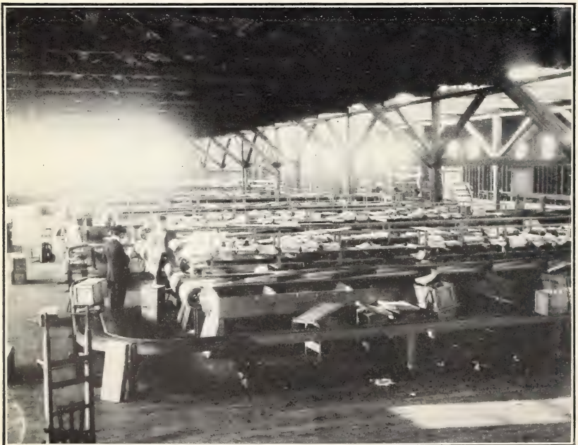
FIG. 2.—GENERAL VIEW OF A CLEAN, WELL-ARRANGED BUILDING.
