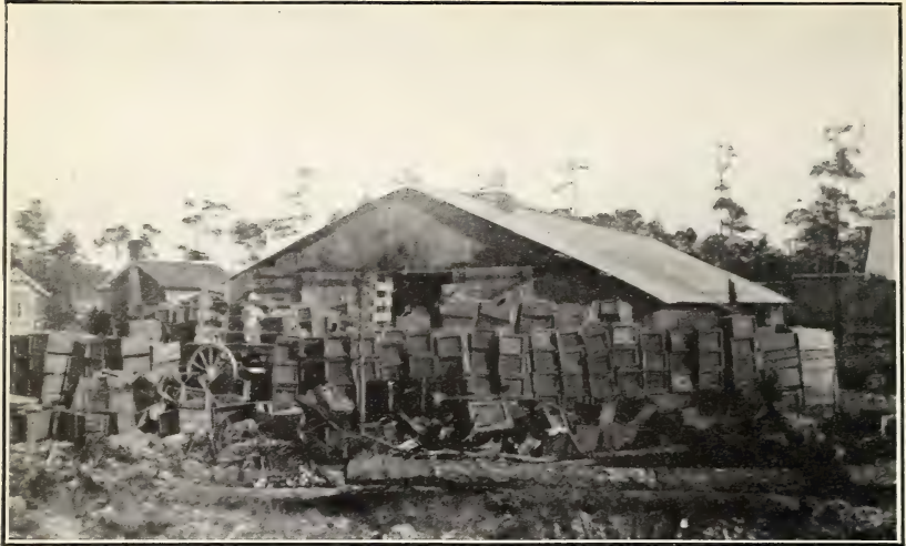
FIG. 1.—AN OLD BUILDING FORMERLY USED FOR PACKING CITRUS FRUITS. Note the crudeness of arrangement, the boxes of grapefruit stacked outside, and the many broken field crates.
