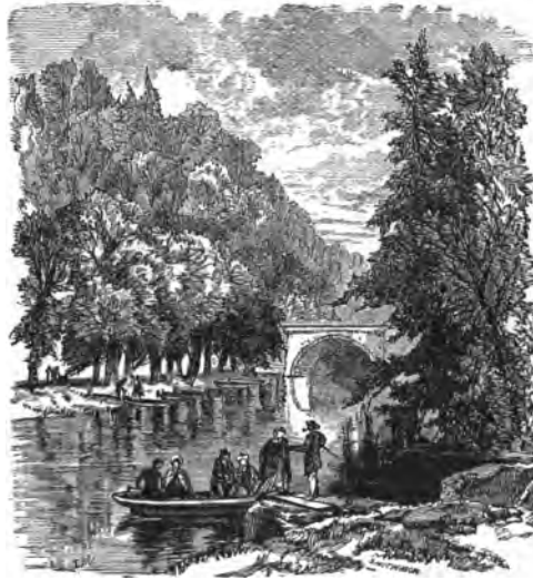
VALLEY GREEN BRIDGE.
