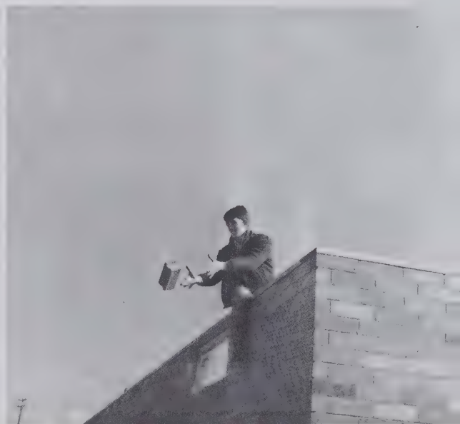
Kenny Revis helps other members work on the field house
