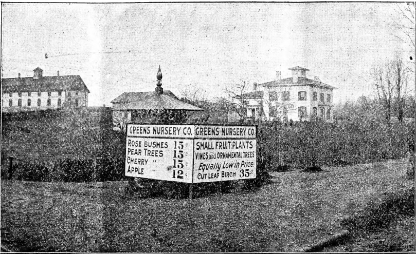
HOME AND OFFICE OF CHAS. A. GREEN AT ROCHESTER, N. Y.
