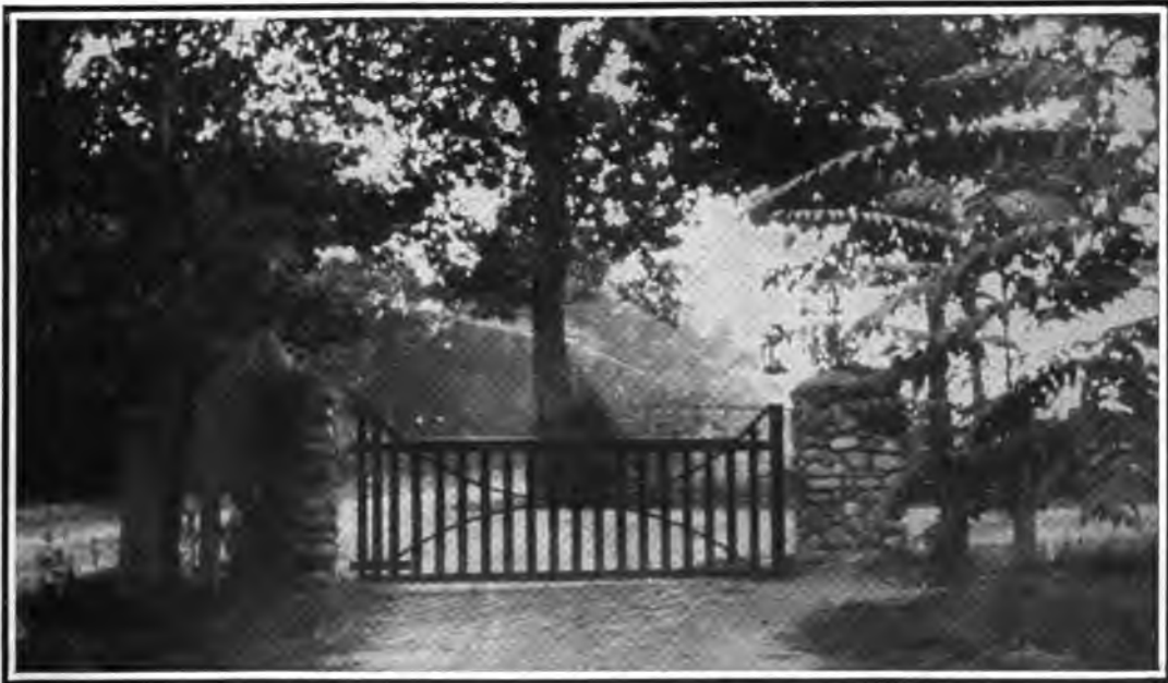
FIG. 388. CONCRETE RUBBLE WORK FOR GATE POSTS.
