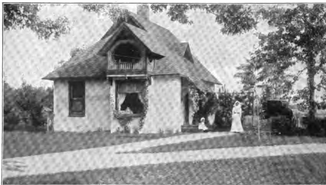
FIG. 399. OUTSIDE PLASTERING OF A FARM COTTAGE.
