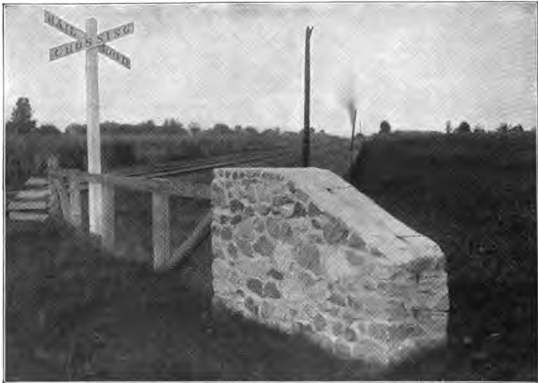
FIG. 480. STONE ANCHOR WALLS FOR FENCE.
