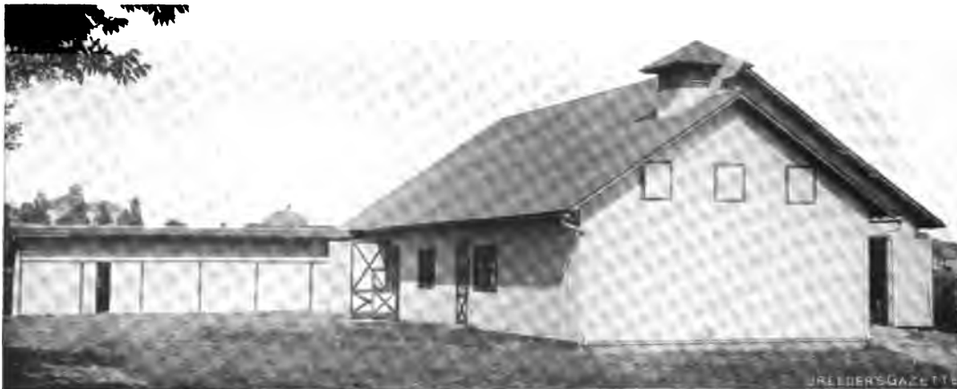
FIG. 246. TENNESSEE DAIRY BARN (SHED ADDITION).
