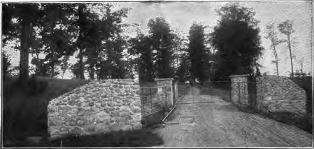
FIG. 479. STONE ANCHOR WALLS FOR FENCE.
