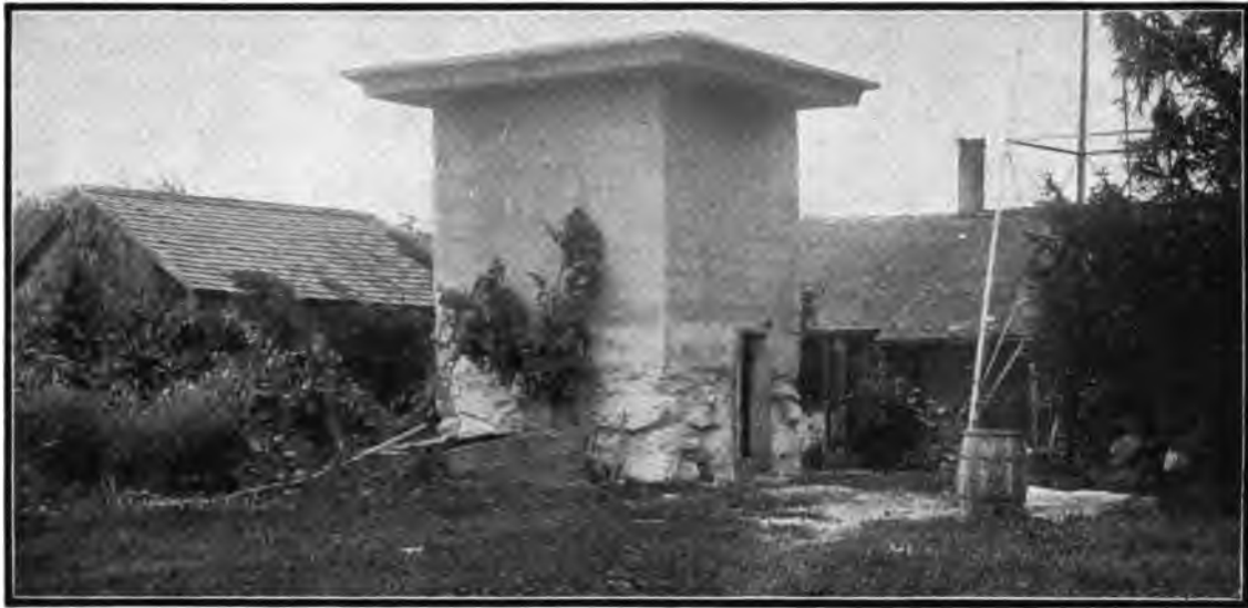
FIG. 394. CONCRETE WATER TANK.
