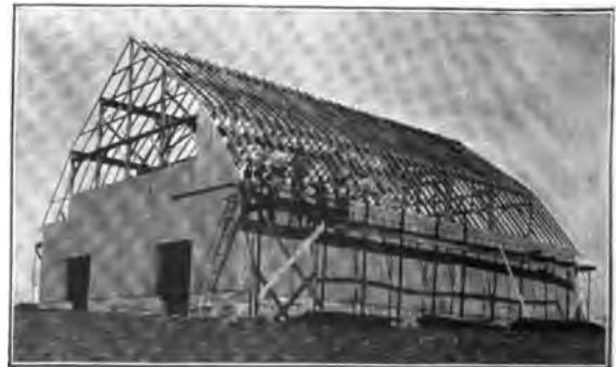
FIG. 108. AN IOWA STEER BARN (CONSTRUCTION).
