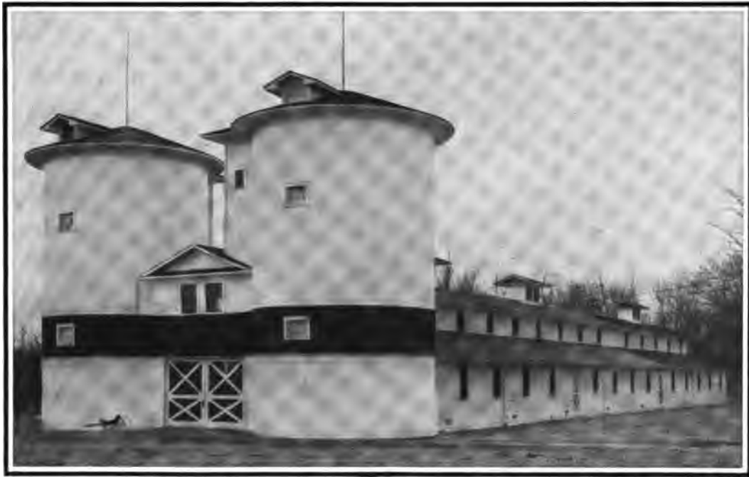
FIG. 405. COMBINATION CEMENT SILO (ELEVATION).
