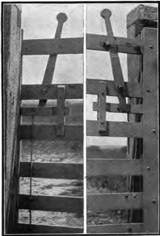
FIG. 525. FARM GATE LATCH.
