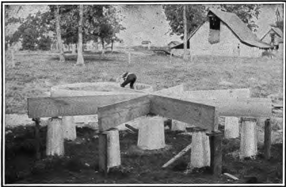
FIG. 421. ROUND RAT-PROOF CORNCRIB (CONSTRUCTION).
