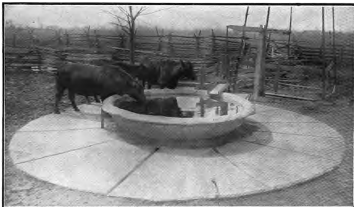
FIG. 398. FARM TANK OF CONCRETE.
