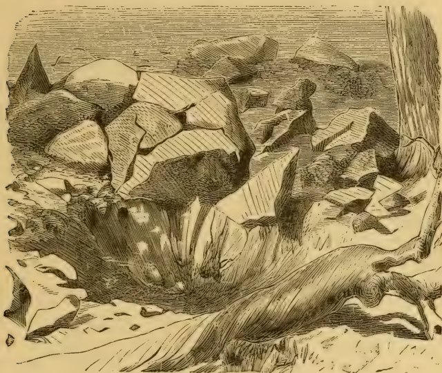
Fig. 46.—THE ROCK AFTER BLASTING.
