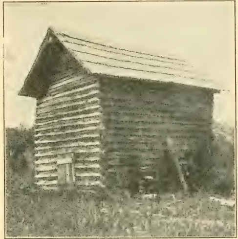
FLUE-CURING BARN, VIRGINIA.
