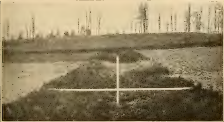
Fig. 16.—A Well-Sodded Surface Run. For convenience and appearance the sides are well sloped and sodded. Seepage water may be removed by a tile laid beneath or at the side of a run like this.
