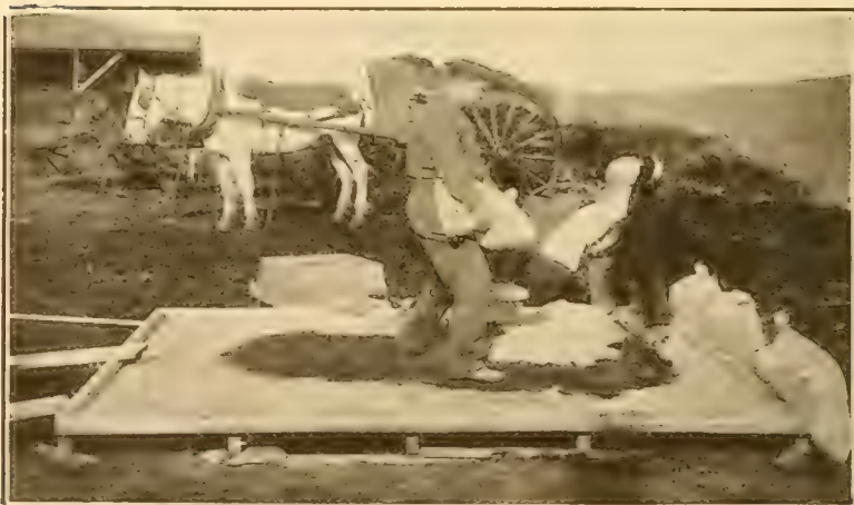
Fig. 3.—Lifting Off the Sand Measuring Box and Getting Cement Ready.
