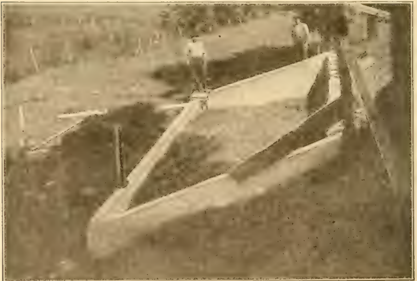
Fig. 33.—Building a Manure Pit in the Side of a Hill.
