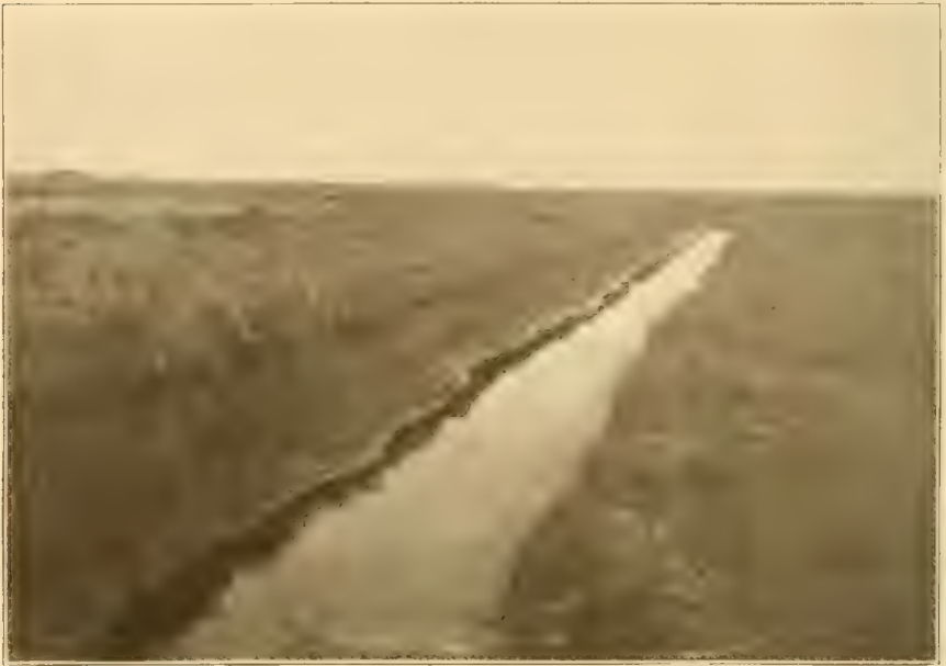
Fig. 6.—An Outlet Ditch. This was dug with a floating dredge, and is 20 feet wide at the top and seven feet deep. Its slopes are somewhat steeper than is advisable. Courtesy of the Wisconsin Experiment Station
