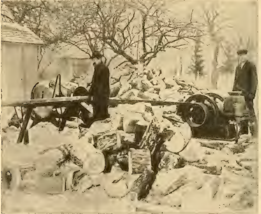
Fig. 1.—Sawing a winter's supply of wood. Select an engine that is large enough for this purpose.
