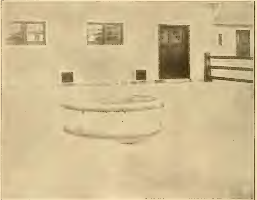
Concrete Feeding Floor and Watering Trough at East Norwich, L. I.
