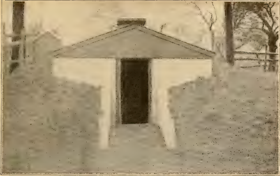
A Concrete Root Cellar.
