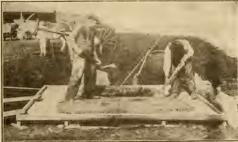
Fig. 5.—First Turning, Sand and Cement.
