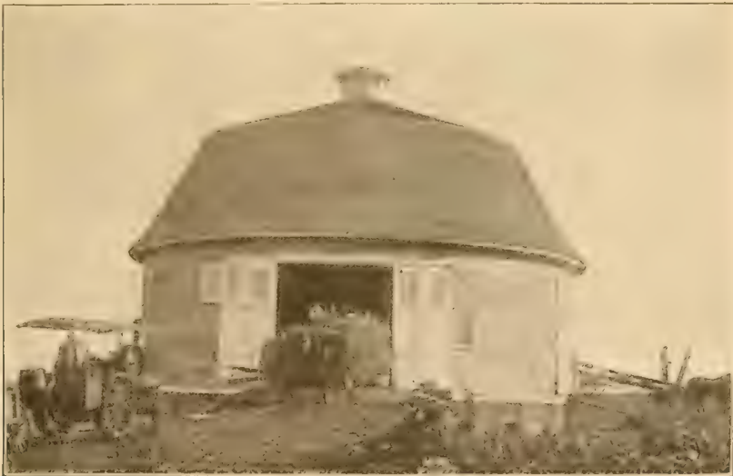
Fig. 21.—The Barn Completed.
