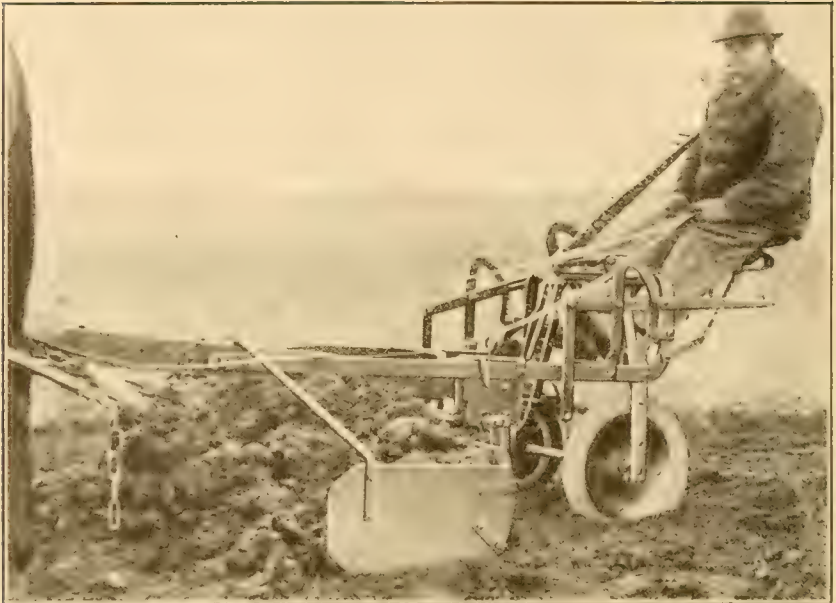
Fig. 9.—A Small Grader being used to transport earth from a high spot to lower ground. It takes the place of the scraper.
