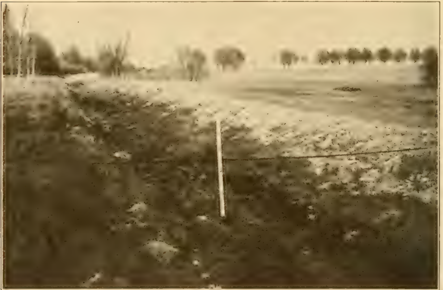
Fig. 17.—A Surface Run with a Dyke on the Side Toward the Marsh. This is only deep enough to serve as an eave-trough to catch the surface water from the adjacent upland. To intercept seepage from the upland a tile has been laid two feet deeper than the bottom of this ditch, and parallel to it, along the edge of the marsh.
