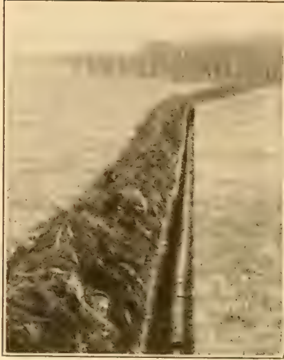
Fig. 11.—Tile Drain Ready to Blind. Courtesy of the Minnesota Experiment Station.
