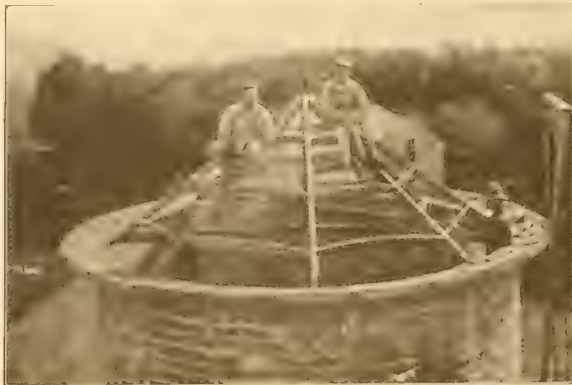
Fig. 8.—False Work and Cornice Block in Place to Receive Sheeting.
