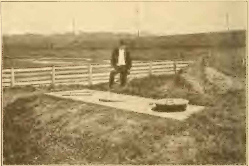
Fig. 37.—Completed Septic Tank.
