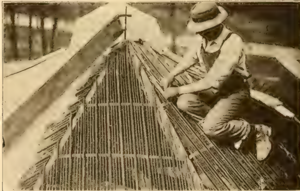
Fig. 28.—Putting expanded metal on false work for concrete roof.
