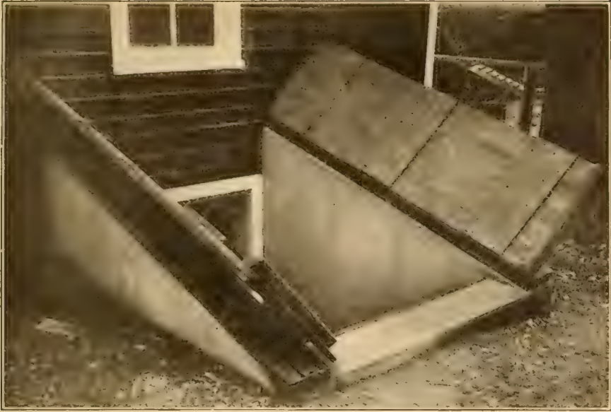
Fig. 38.—Concrete Cellar Way.
