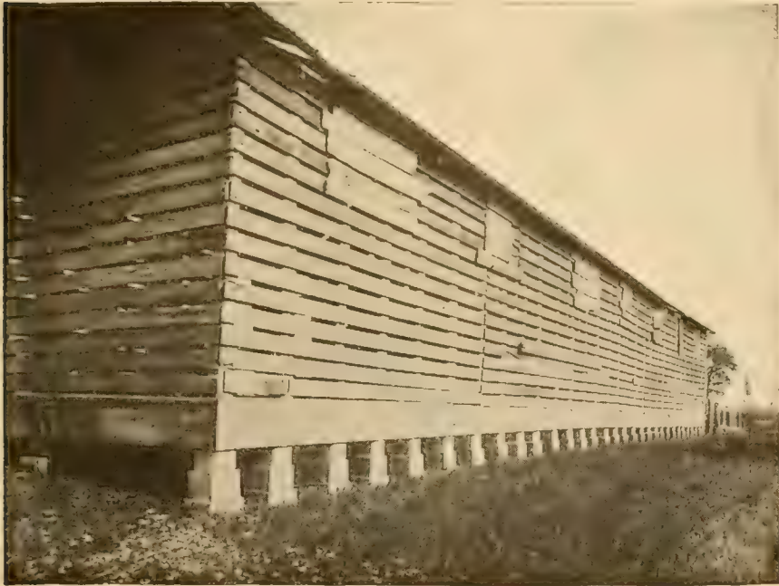
Fig. 22.—Concrete Pier Supports for a Large Corn Crib.
