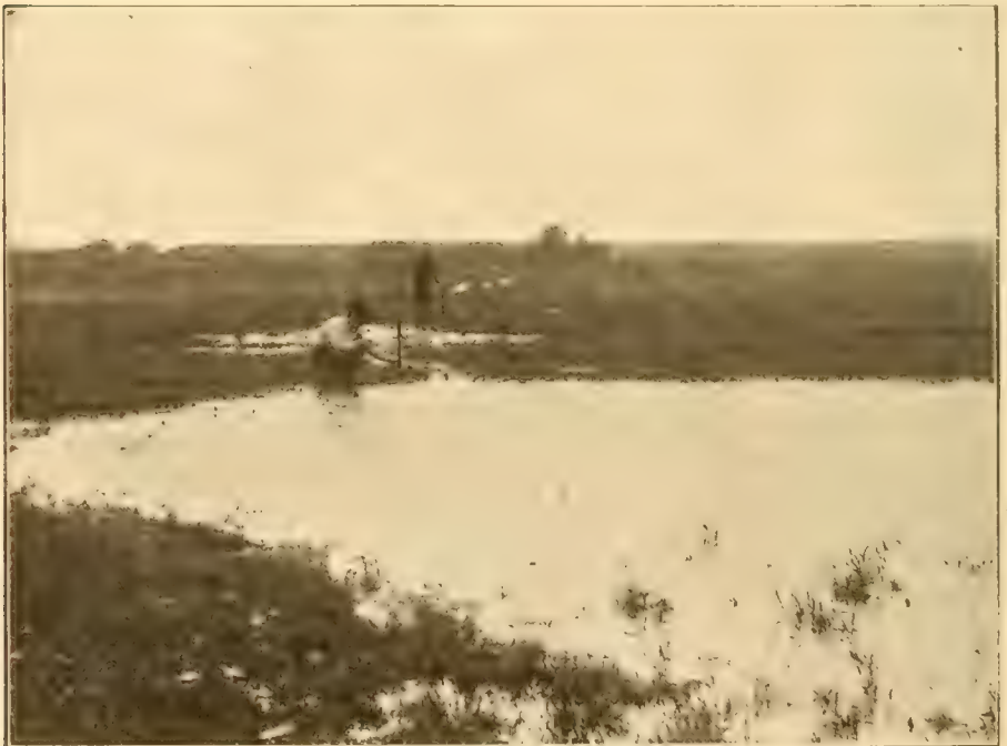
Fig. 4.—Operating a Leveling Instrument.
