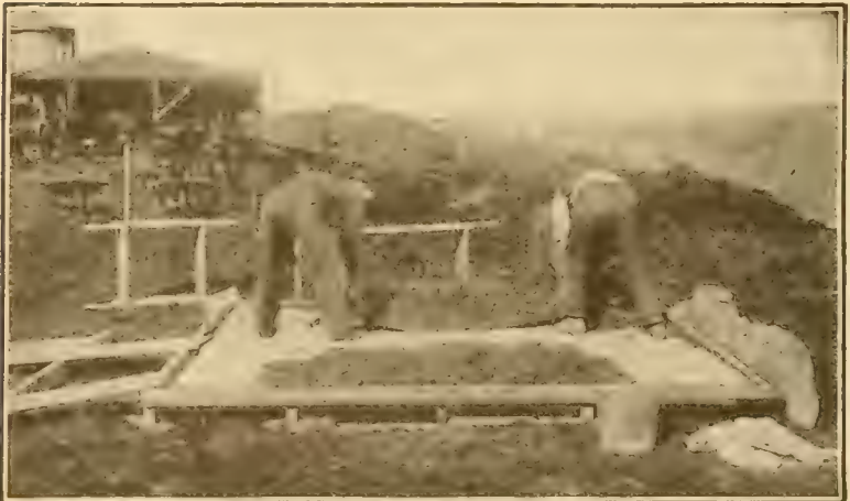
Fig. 10.—Mixing the Stone (or Gravel) With the Sand and Cement.
