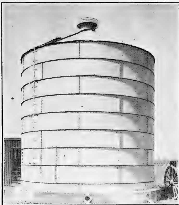
FIG. 16.—A modern galvanized-iron corncrib planned and erected by a progressive dairyman of Louisiana. Soft white dent corn has been kept in this crib in perfect condition for over a year. Weevils breed in such cribs as fast as in any, but are easily killed by fumigation with carbon disulphid. (Photograph by Jones.)
