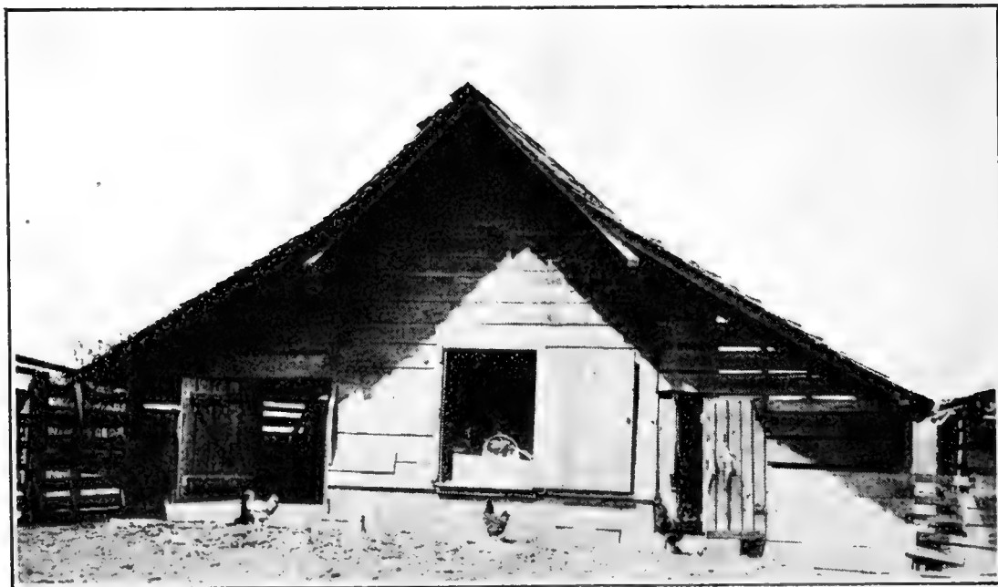
FIG. 15.—An old-style barn with lean-to sheds. The owner could not store corn or wheat and keep it free from weevils. At the advice of the county agent he sealed the barn on the inside with tongue and groove boarding, and filled the space between the rough outer boards and sealing with packed sawdust. He then fumigated with carbon disulphid and killed all weevils. Use your ingenuity to tighten your old crib or build a new one, according to the advice of your county agent.
