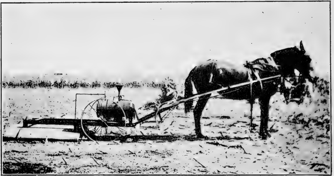
FIG. 14.—Five-torch asphalt heater adapted for burning chinch bugs.
