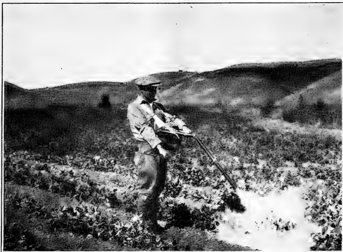
FIG. 6.—Hand-operated fan duster in use against the pea aphid.
