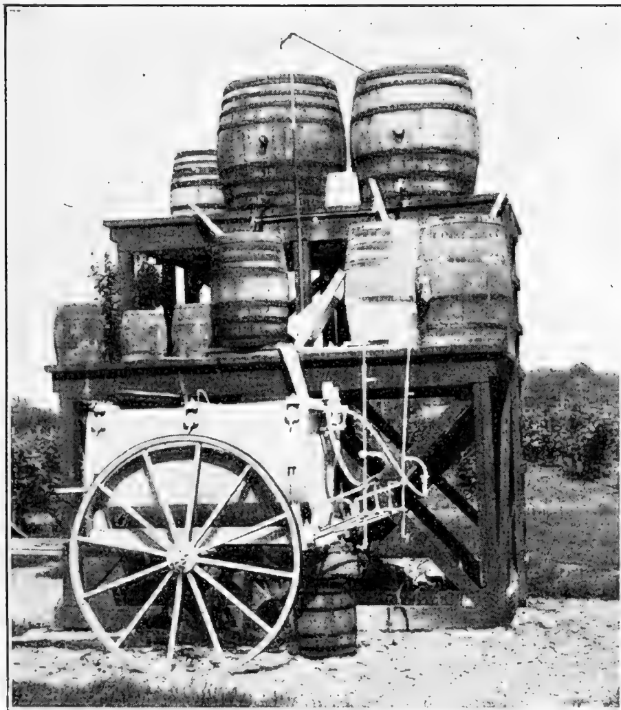
FIG. 72.—Bordeaux mixing plant.
