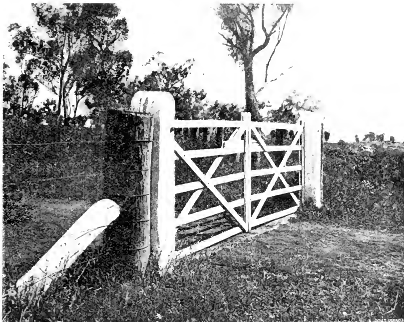
Fig. 13.—A gateway with squared and trimmed posts.
