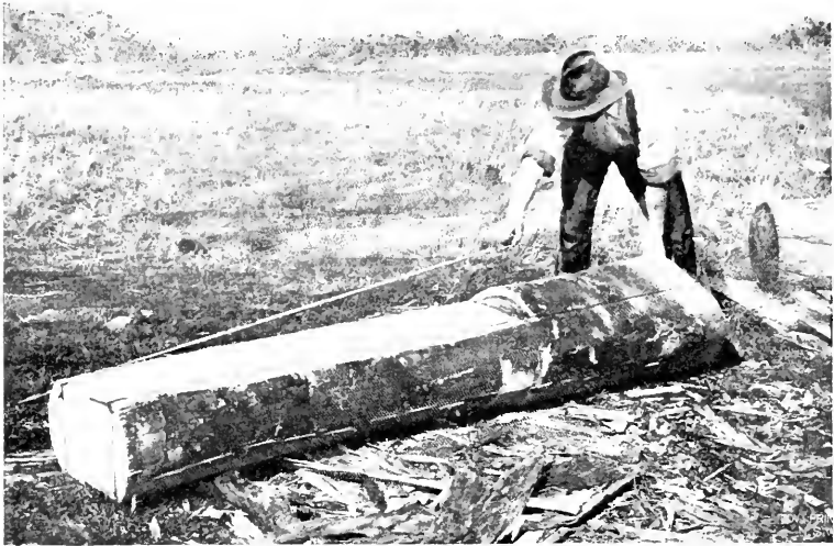
Fig. 20.—Striking after the first two edges have been squared.
