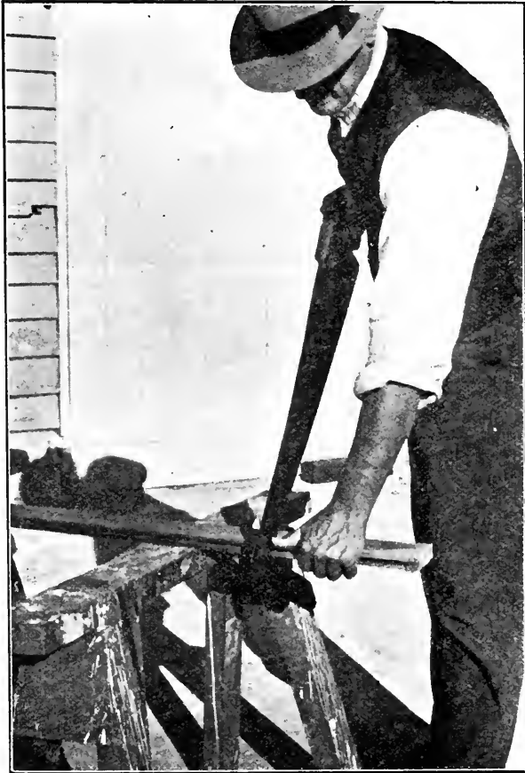
Fig. 21—The Correct Use of the Saw.
