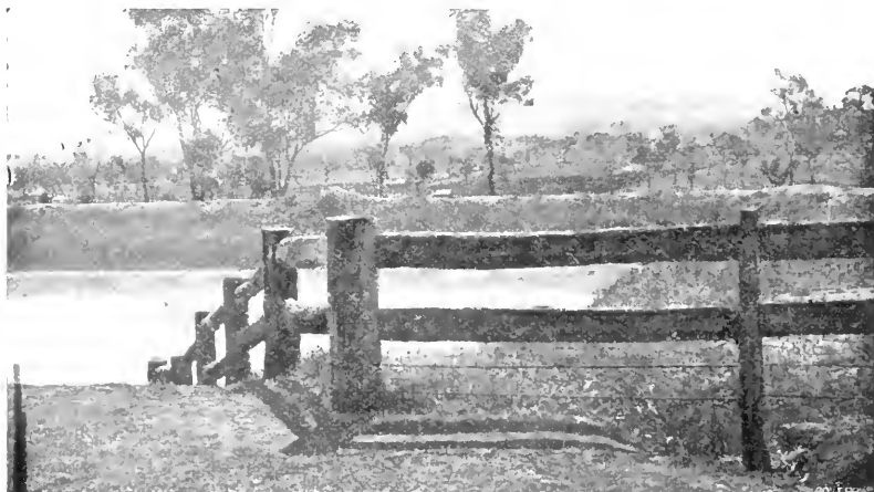
Fig. 5. A two-rail fence with two wires.
