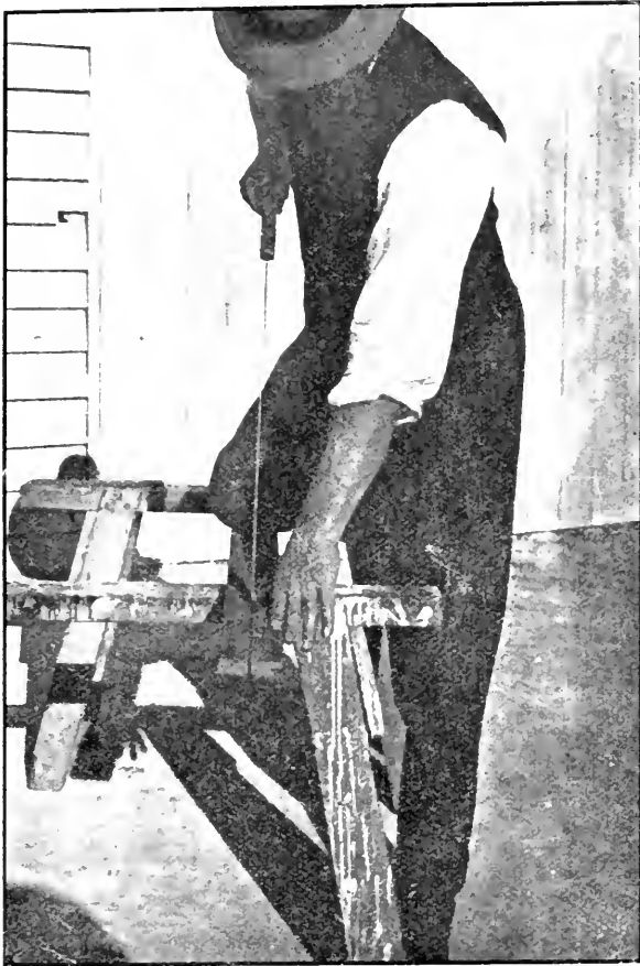
Fig. 23 The Correct Use of the Saw. Keep the arm-pit plumb over the saw-cut.
