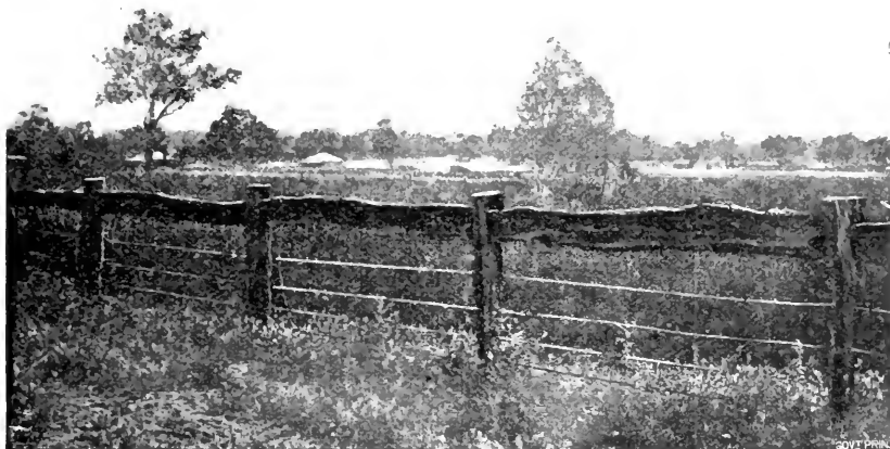
Fig. 6.—Top-rail and wire fence; eight posts per chain.
