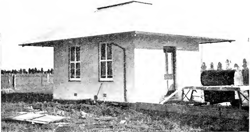
Fig. 22.—A small dairy built of ash concrete. Note the neat and solid appearance.
