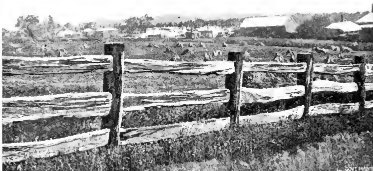
Fig. 4.—Three-rail fence; eight panels per chain.
