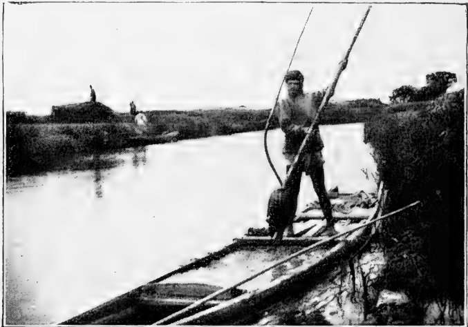
FIG. 88. — The young man is loading his boat with canal mud, using the long-handled clam-shell dredge; which he can open and close at will.
