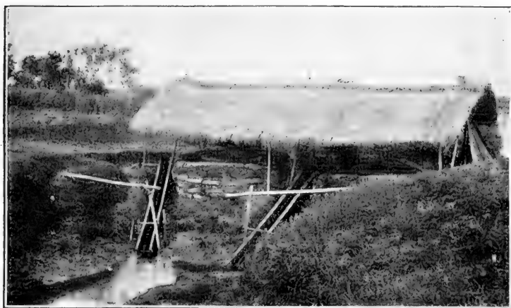
FIG. 140. — Pumping station on the farm of Mrs. Wu, showing pump shelter, two power wheels connected with pumps, set at the end of a water channel leading from a canal.
