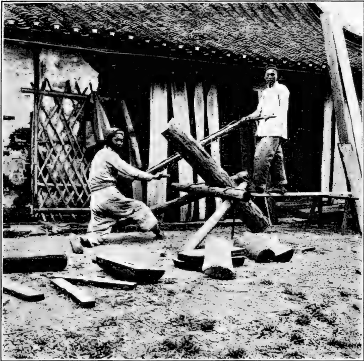
FIG. 28. - Usual method of sawing lumber in China.
