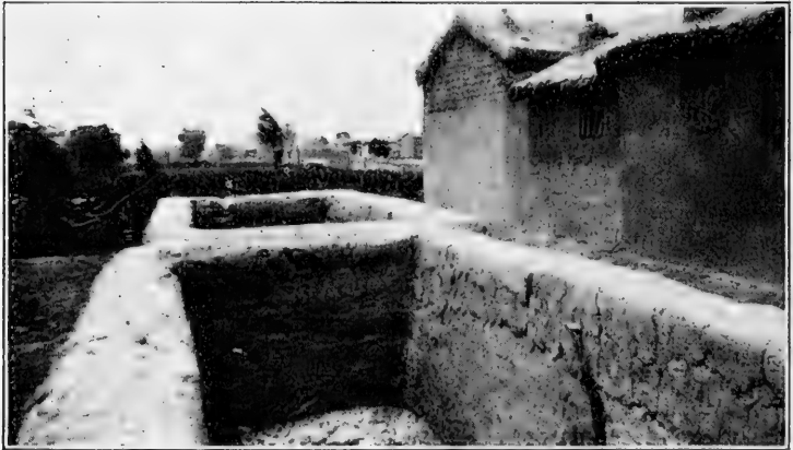
FIG. 73. — Millet-thatched roofs plastered with earth; mud chimneys; walls of houses plastered with mud, and winter storage pits for vegetables built of clay and chaff mortar.
