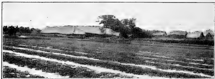
FIG. 139. — Residence compound and farm buildings of Mrs. Wu, Kashing, China.
