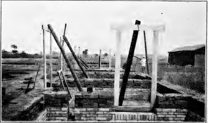
FIG. 75. — Foundation of dwelling, consisting of hard-burnt brick; balance of wall to be sun-dried earth brick, seen in Fig. 74.
