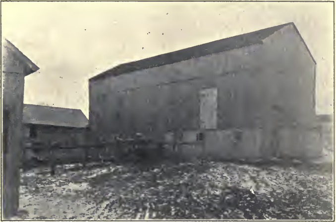
FIG. 102. — The dairy barn on the farm given on page 537. Over 75 years old, but serviceable and economical. See Figure 103.
