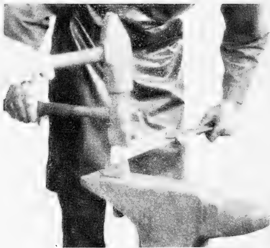
FIG. 243. Using the fullers.
