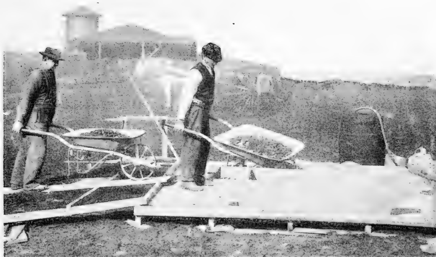
FIG. 138- a . Measuring coarse aggregate.
