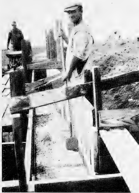
FIG. 141. Working stones away from surface.
