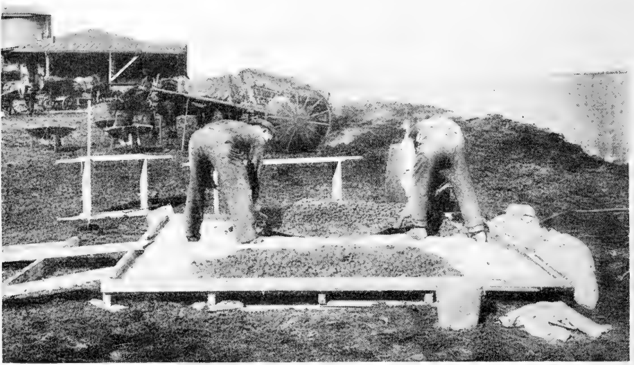
FIG. 139- a . Turning the mixture.
