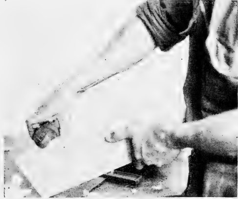
FIG. 27. Correct method of holding gage and stock.
