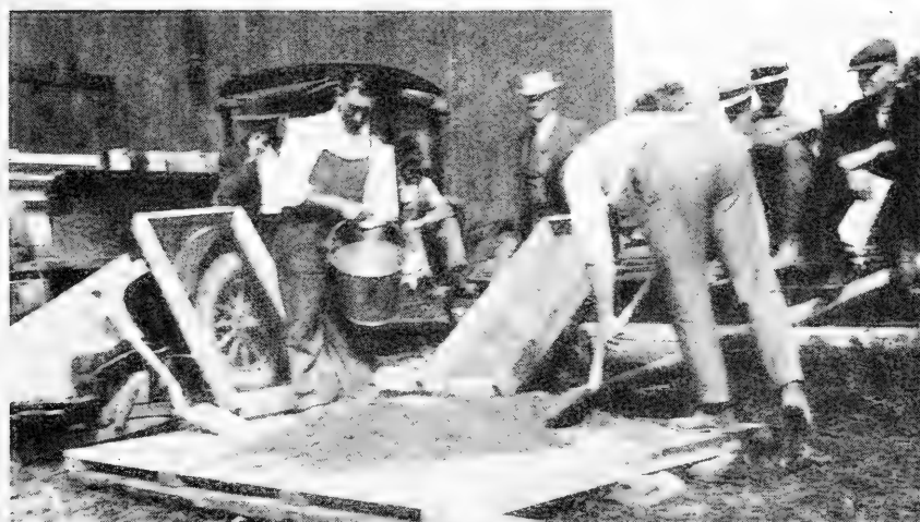
FIG. 139. Adding water to mixture.
