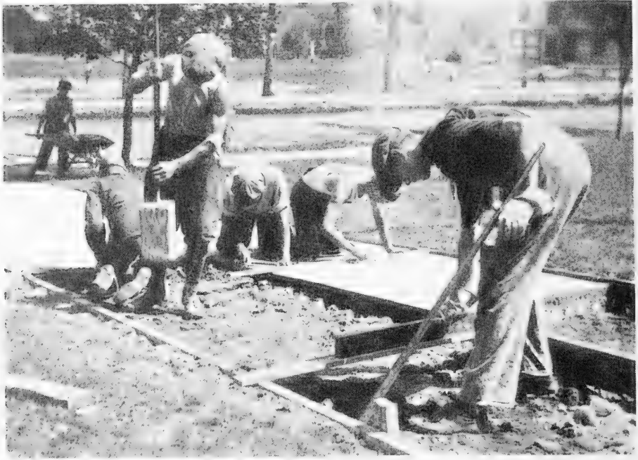
FIG. 148-a. Boys constructing sidewalk.
