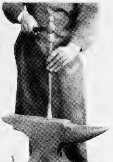
FIG. 208. Upsetting for two-piece weld.
