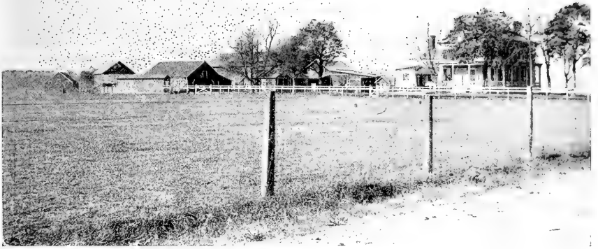
Fig. 2.—A Typical Group of Farm Buildings in Monmouth County, New Jersey.
