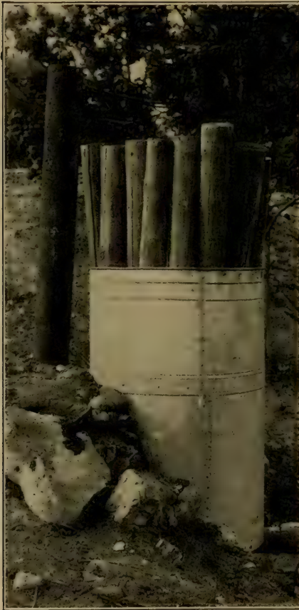
FIG. 55. — Single tank for treating posts.
