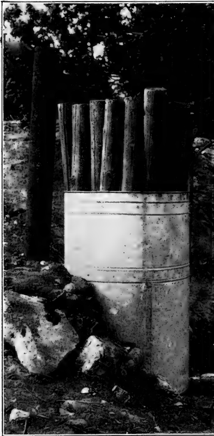
FIG. 55. — Single tank for treating posts.
