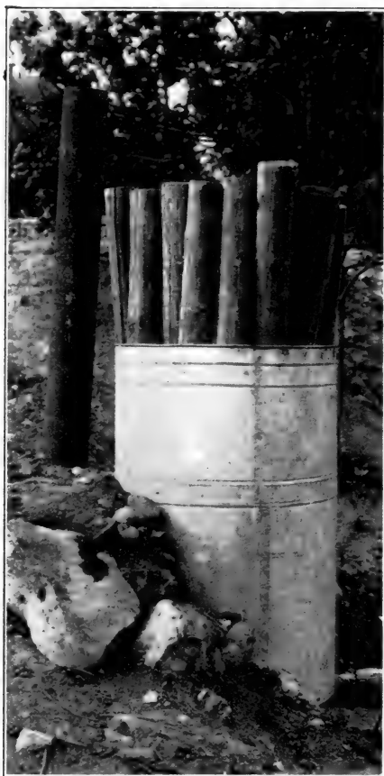
FIG. 55.—Single tank for treating posts.
