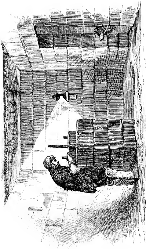
Interior of the Magnetic Observatory.
