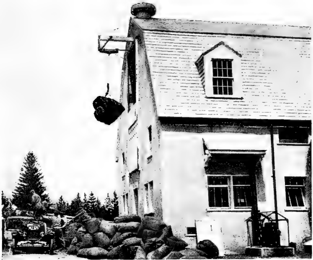
HOISTING MACHINERY IN OPERATION
