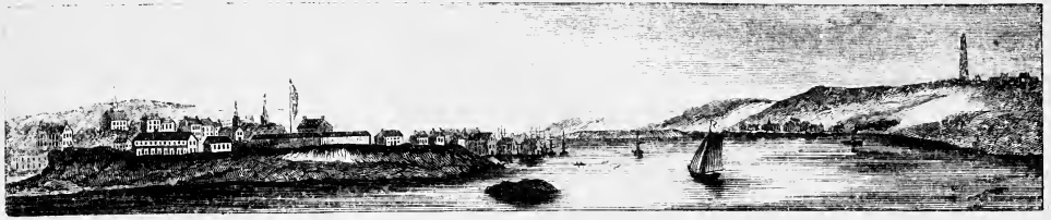
NEW LONDON HARBOR, LOOKING NORTH. 2
