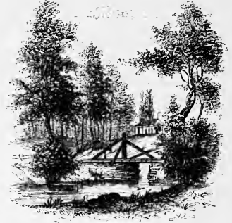
BRIDGE OVER SLEEPY HOLLOW CREEK.
