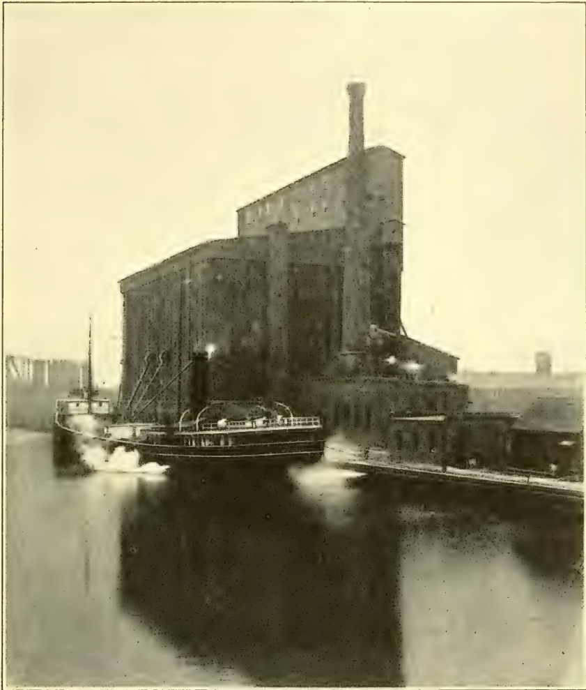
FIG. 132. — A terminal elevator in Chicago located so as to ship grain by rail or boat.
