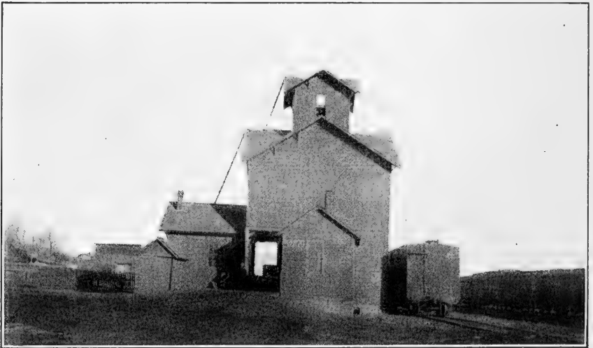
FIG. 131. — A typical country elevator.
