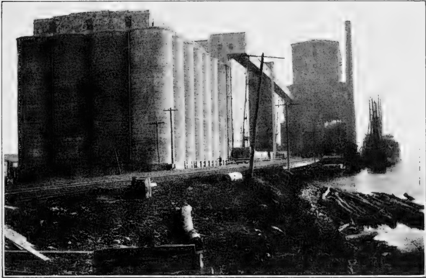
FIG. 134. — An elevator and concrete storage bins at Baltimore, Md. Grain is exported from here.
