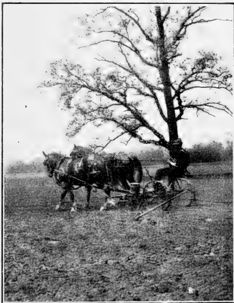
FIG. 21.—Planting corn with a check rower.
