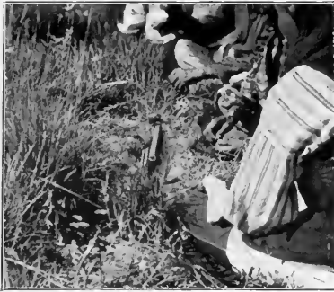
FIG. 19. The pipe-tampers and new earth.
