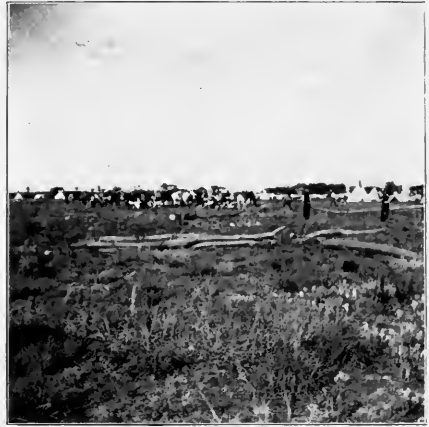
FIG. 43. Preparing the timbers for the lodge.
