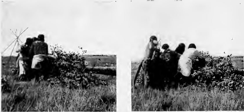
FIG. 51. Placing the brush in the fork of the center-pole.
