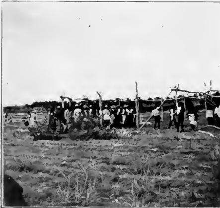
FIG. 44. Erecting the lodge.
