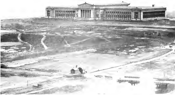
About 1920. What must have been a sea of mud surrounds the completed Museum. The underground railway (shown above) has been covered. Landfill extending into Lake Michigan is still to be added on three sides of the building.
