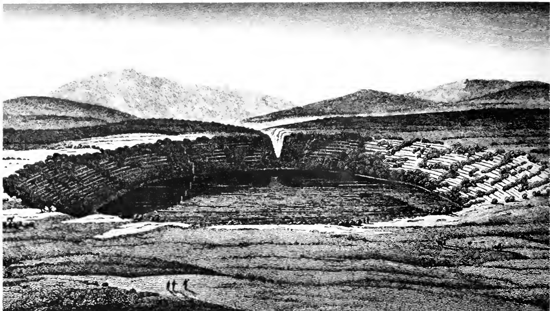
Lake Guatavita, showing the results of Antomo de Sepúlveda's attempt to cut through the enclosing rock and thus drain the lake. Begun in the 1580s, the project employed some 8,000 Indian laborers but was eventually abandoned. From an 1810 engraving.
