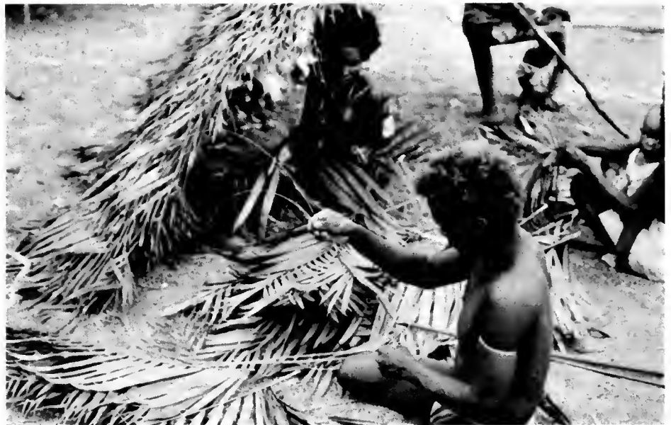
An Agta couple work together in the construction of their lean-to shelter. As he prepares cord from plant fiber she uses the cord to attach shingles.
