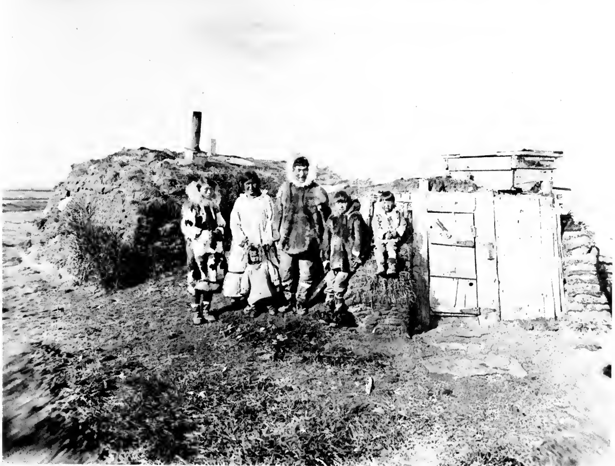
Chief reindeer herder at Point Hope, Alaska, with his family outside semisubterranean house. Note the use of sod blocks. Courtesy the Archives and Historical Collections, the Episcopal Church. 29
