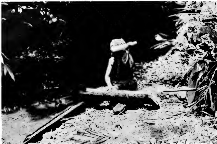
An Agta couple work together in the construction of their lean-to shelter. As he prepares cord from plant fiber she uses the cord to attach shingles.
