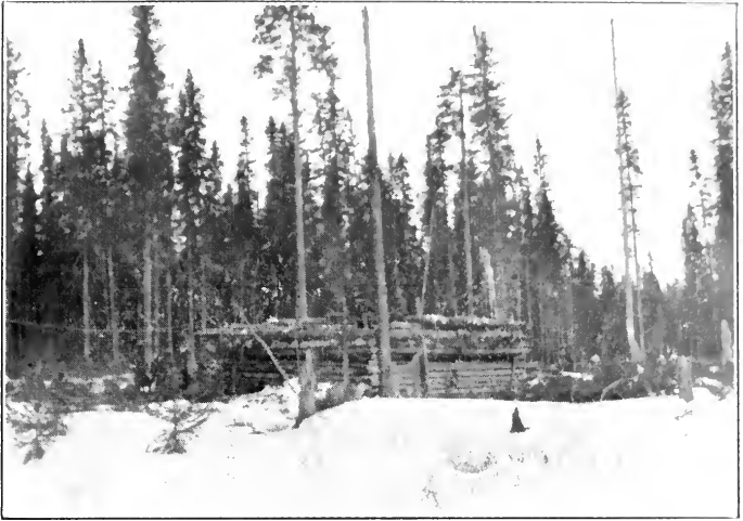
The American Engineers built scores of block houses like this.
