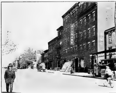
South Portland Avenue—Storage warehouse and stables near private houses.
