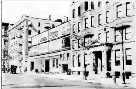
Cathedral Parkway, near Seventh Avenue—Garage opposite Central Park and in a high-class apartment house district.
