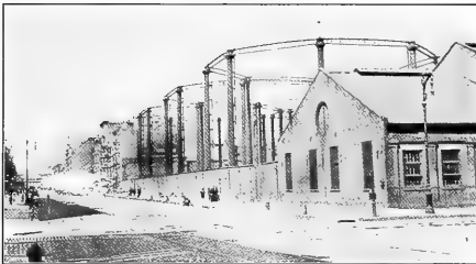
East 14th Street, Between Avenues B and C—Gas tanks next and opposite to tenements. Note tenement children playing near them.
