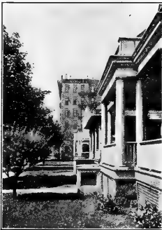
East 19th Street, near Cortelyou Road, Flatbush—Apartment house in exclusive private house district.
