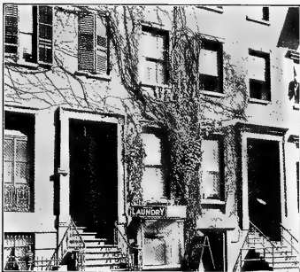
West 8th Street—Basement of private house converted into public laundry.
