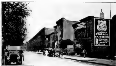
1191 Bedford Avenue—Garage near private homes.
