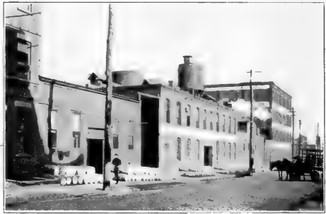
North 11th Street, Williamsburg—Barrels of paint stored on the sidewalk for the entire length of block.
