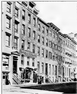
West 8th Street, between Fifth and Sixth Avenues—Conversion into stores.
