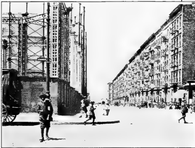
West 66th Street and Amsterdam Avenue—Gas tanks in tenement house district.
