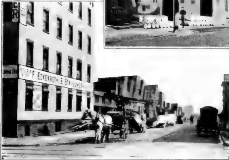
East 5th Street, near Lewis Street—Lumber yard and planing mill. Note lumber stored on sidewalk and roadway.
