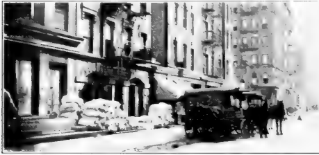
339 East 107th Street, near First Avenue—Wet wash laundry next to tenement.
