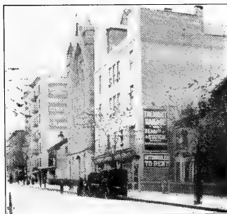
Washington Avenue, near Tremont Avenue—Garage between a private house and a church.
