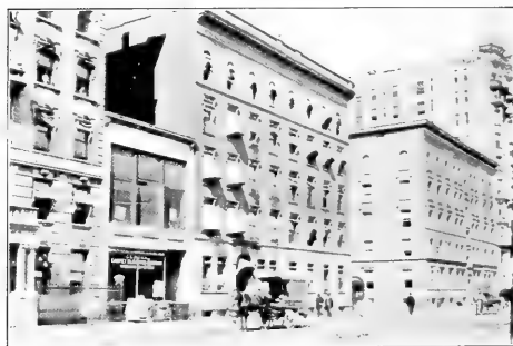
Central Park West and 98th Street—Loft building and carpet cleaning works.
