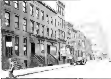
East 10th Street, west of Third Avenue—Converted private houses
